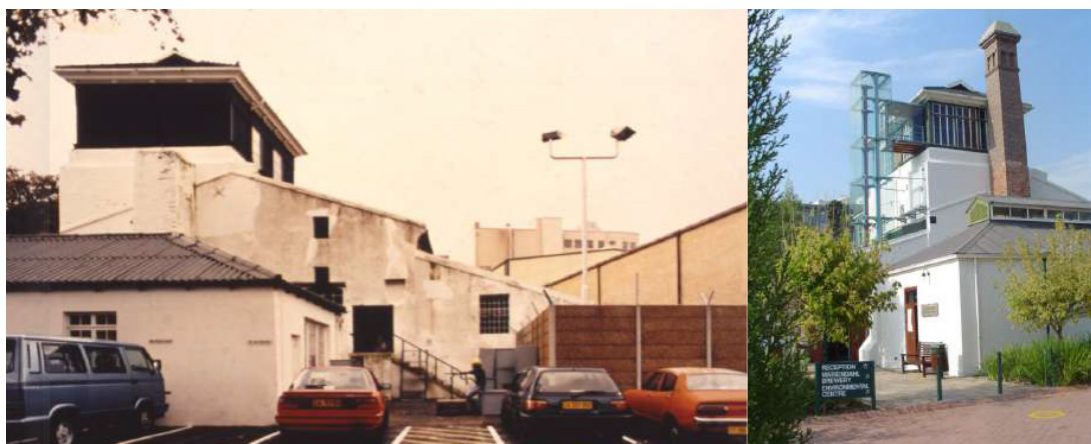
Figure 7 Visitor's Centre for the South African Breweries (SAB), Newlands, Cape Town. Left: original brewery (1859-1903) (source: courtesy Fagan archive). Right: Visitor's Centre with new lift and extended chimney (photograph by the author, 2007).
