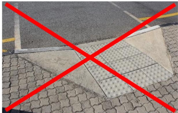
Figure 2: Old Standard Tactile Pedestrian crossing
