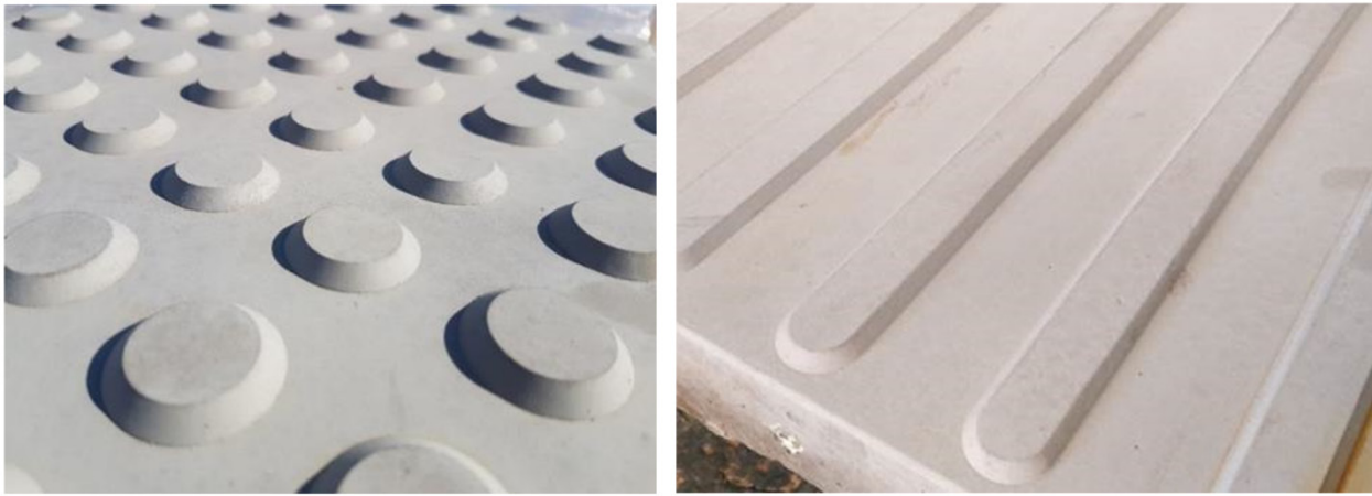
Figure 5: Correctly manufactured SANS 784 Warning and Guiding Tactile Blocks
