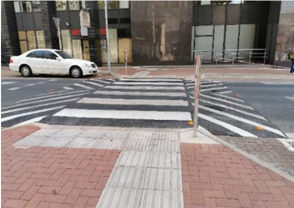
Figures 13: Controlled, L-Shaped raised Tactile Pedestrian Crossing
