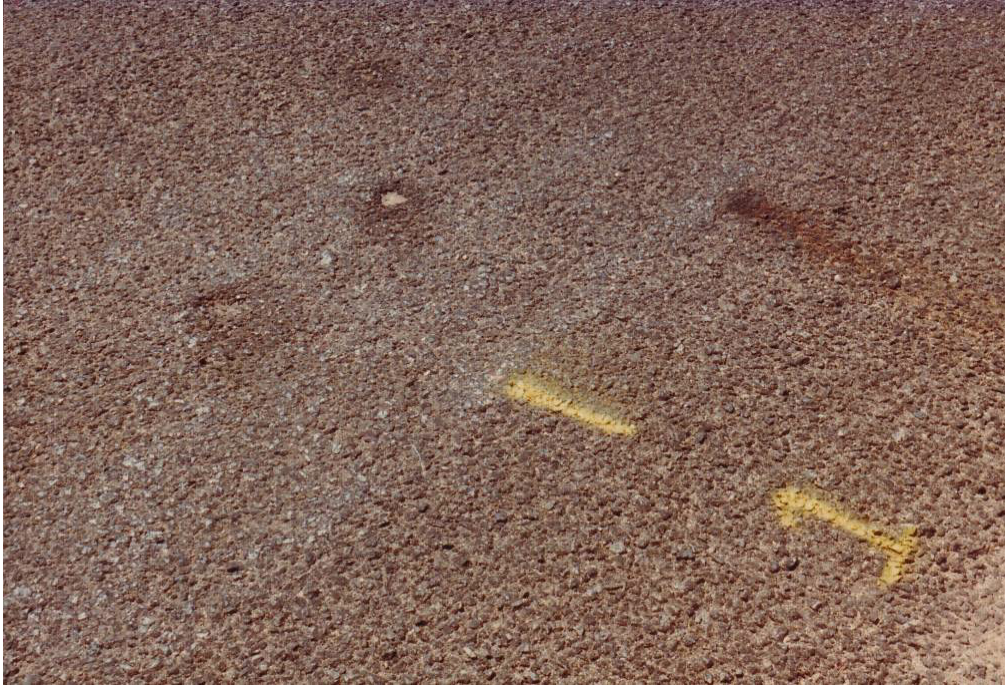
Figure 5: Cratered blisters and brown staining on 1980 13 mm reseal at km 19,997: Average diameter 60 mm, depth 15 mm, spacing 400 mm (TOSAS photo)
