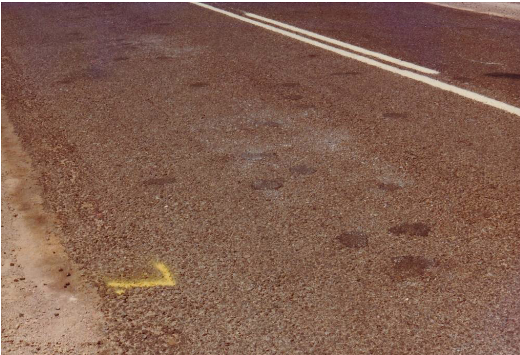
Figure 6: Craters on 1980 13 mm reseal pre-patched with slurry and blisters flattened with steel-wheeled roller at km 19,540 (R) for bitumen-rubber Section 12: Average spacing 400 mm (TOSAS photo)
