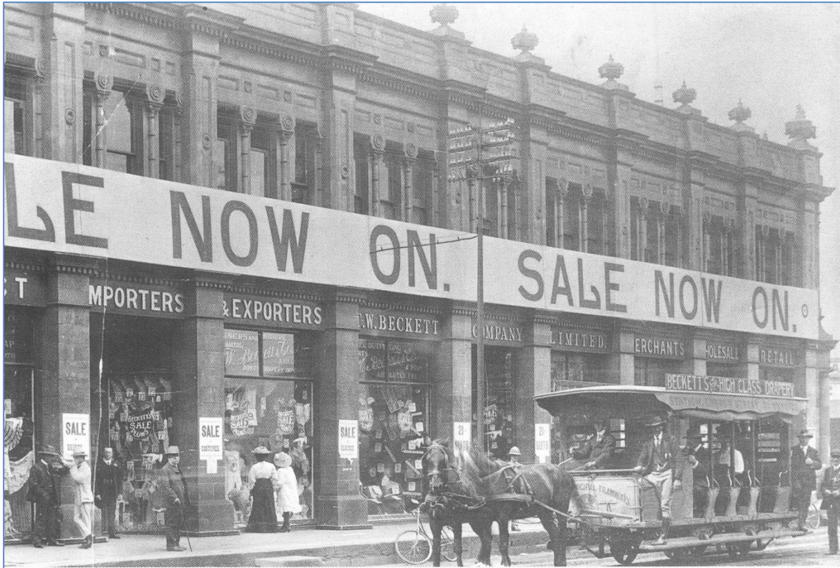
Figure 6: Tom Beckett's store on the corner of Church and Van der Walt Streets in 1910. A horse drawn tram and commercial patrons are visible in this very busy area (Allen 2007: 144).
