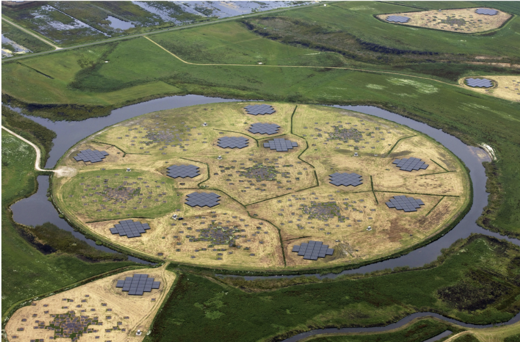
FIGURE 1.13: The LOFAR core. In the upper right and lower left of corners of the three additional LOFAR cores stations can be seen. Each of these core stations includes a field of 96 LBAs and two sub-stations of 24 HBAs each (van Haarlem et al., 2013).
