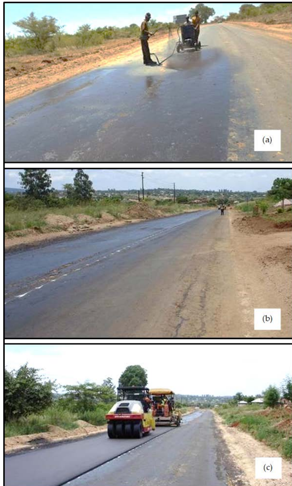
Figure 13. (a) Hand application of a quick-drying anionic-diluted NME prime coat to protect the base before application of the surfacing; (b) application of a tack coat 2 months after construction of the base-layer (opened to traffic); and (c) application of the surfacing. Note the little damage to the base-layer after two months open to traffic during the holiday and rainy season.
