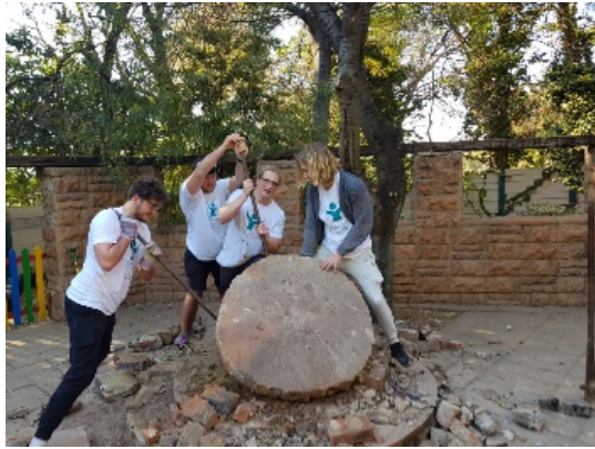
Figure 4: Group 195 lacked the equipment to move a heavy slab Source: The photograph was submitted on the LMS by Group 195 of 2019
