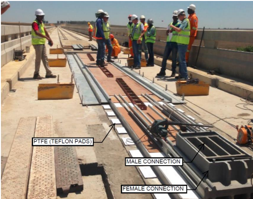
Figure 3.8: Construction of Stage 3 PY Track Slab
