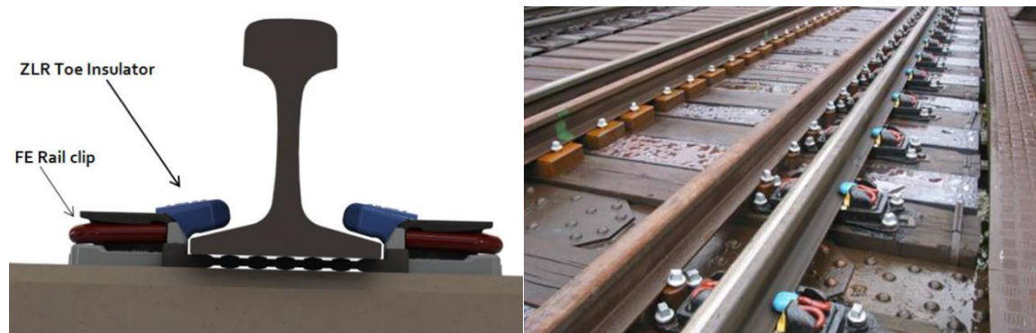
Figure 2.11: Example of ZLR's installed on rail bridge
