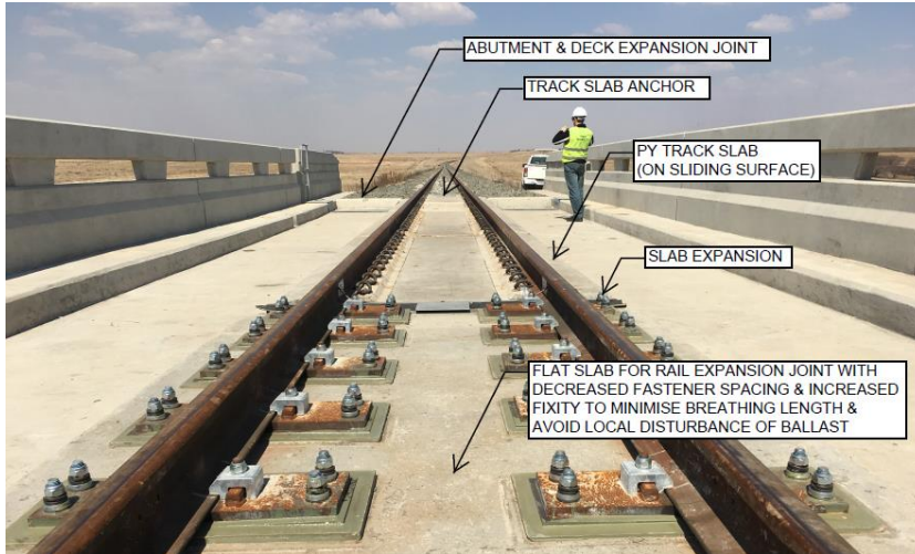
Figure 2.10: Rail Expansion Joint (Photograph: Transnet Capital Projects)
