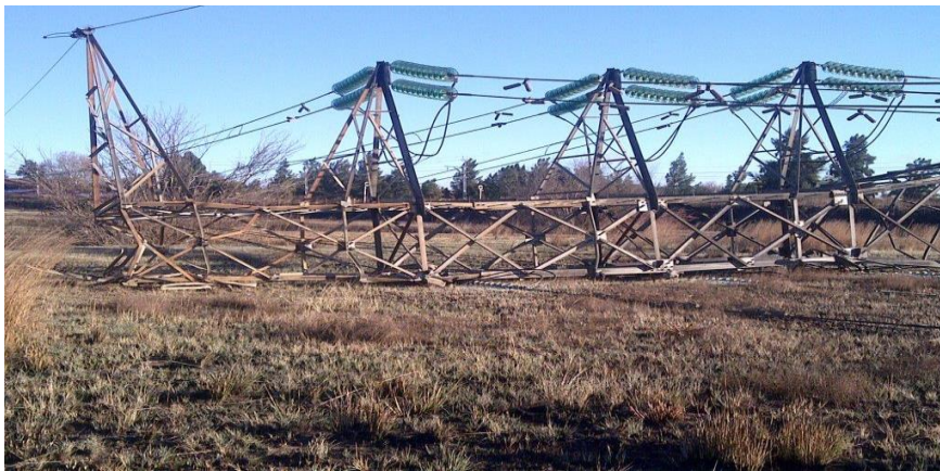
Picture1. Cable theft in Springs on the 5 th June 2014
