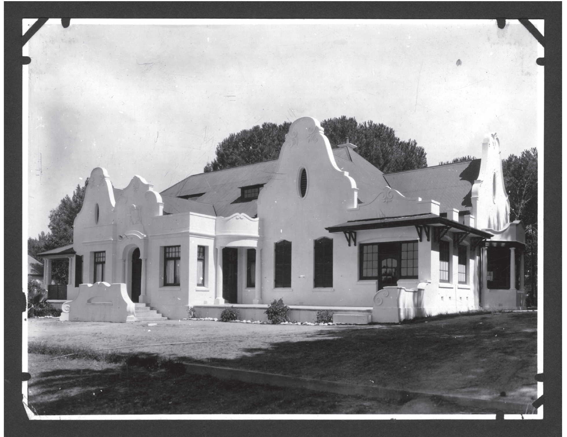
Fig. 1.1 A house designed by Mello Damstra featuring gables in the Cape Dutch Revival style, a recurring feature across his wide range of residential projects in the broader Cape region.
