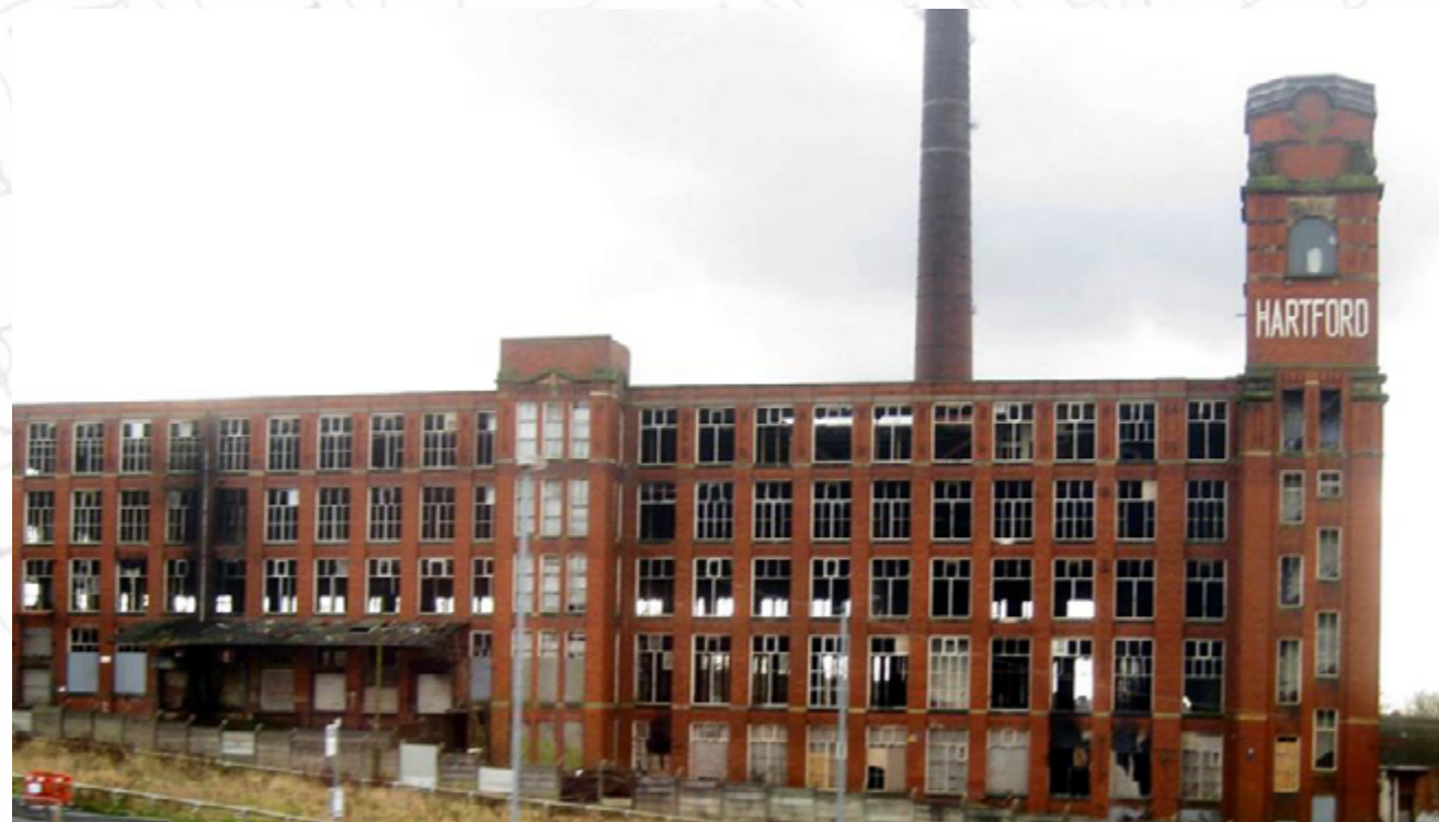
FIGURE 22 - Derelict Light Industrial Building (Diego Sunburns, 2021)
