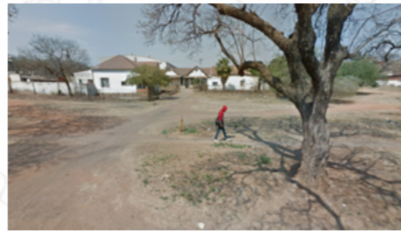
2 FIGURE 30 - OLD HOUSES AROUND SITE (GoogleMaps, 2017) DERELICT - DISCONNECTED
