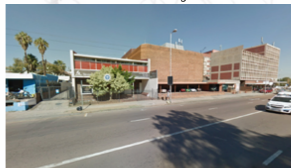
9 FIGURE 37 - MULTI STOREY RESIDENTIAL (GoogleMaps, 2017:online) BLANK FACADES
