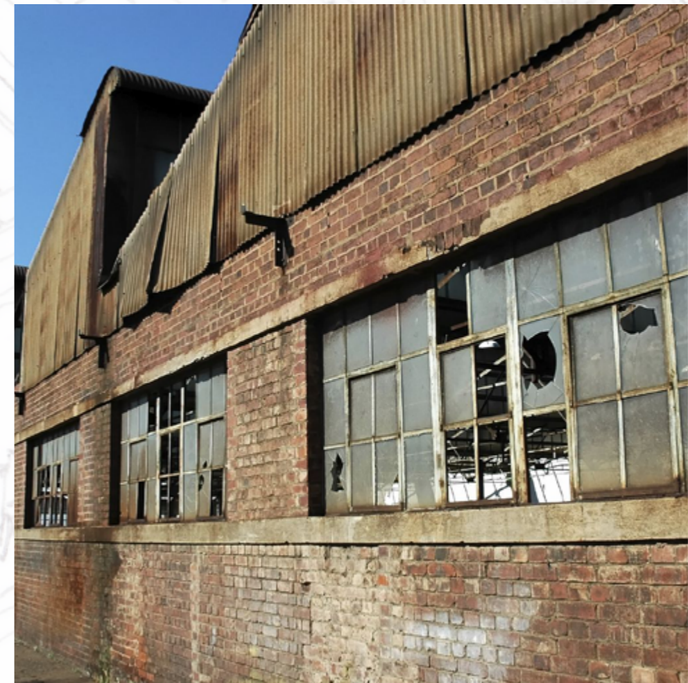
Figure 7 - Old Light Industrial Building (S.Dadlei, 2020)
