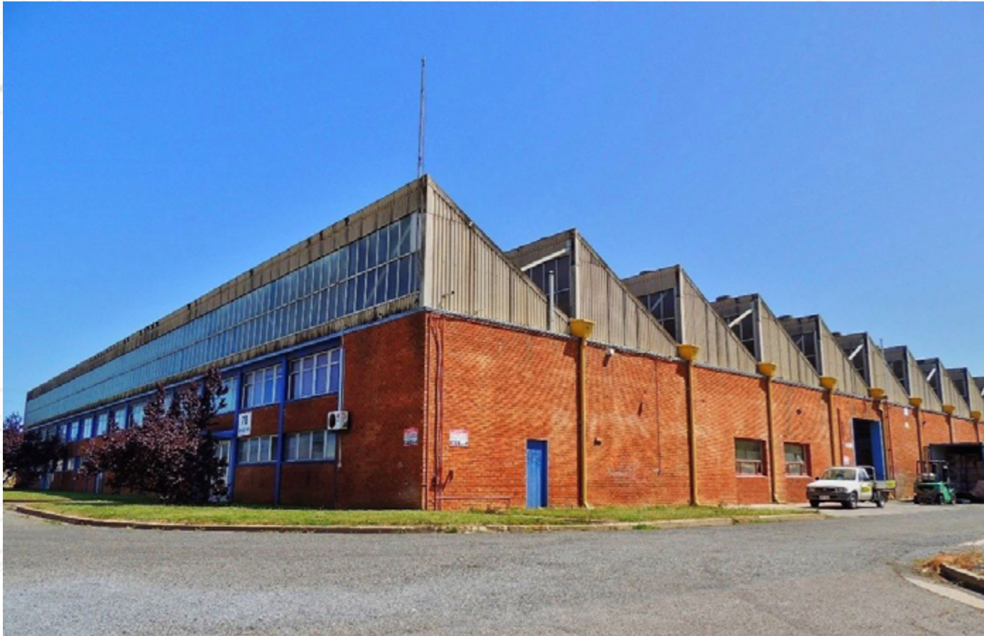
FIGURE 98 - Typical Light Industrial Building (Valles, 2021)
