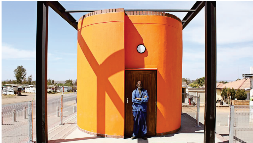
Photograph showing amenity buildings sitting separate from the frame structure. (New Urban, 2016)
