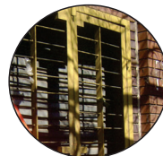
Steel Frame Shutters
