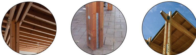
1. Timber Framing. Timber profiles will be used to cover some of the steel columns as a design feature
