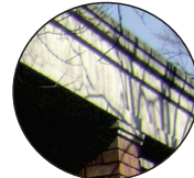
Concrete Up-stand Beams
