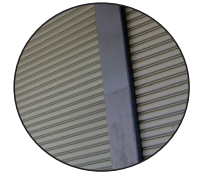
Steel Sheetting facade infill steel frame
