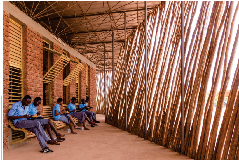
Fig 94: Photograph of intermediary space between the eucalyptus wood screen and classroom walls (Kere Architecture 2019)
