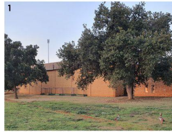
1 Western facade of the squash courts: Solid, inaccessible wall.
