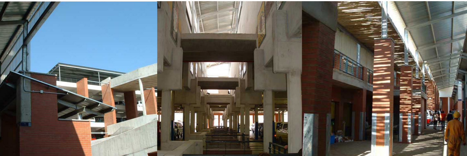
Figure 5.26-5.28 The grand double-volume entrances orient the users, while robust, hard-wearing materials such as red facebrick and off-shutter concrete provide a feeling of structural permanence and durability (Artefacts 2002).
