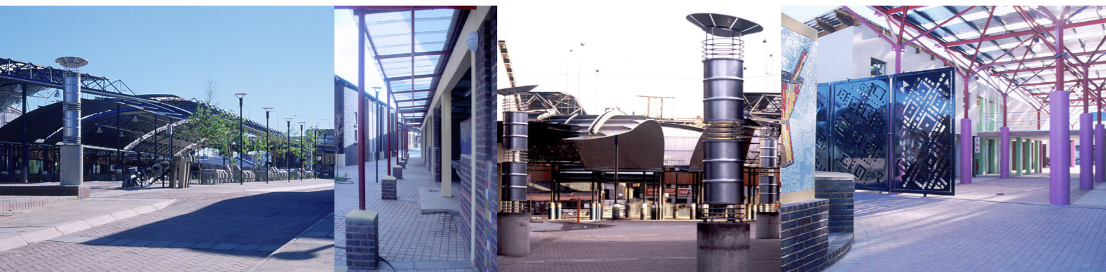
Figure 5.18-5.21 The wave-like corrugated iron rooftops and steel girders allow for increased natural light to fill the spaces below, and are juxtaposed by the angular shape of the factories and markets (MMA Design Studio n.d.).
