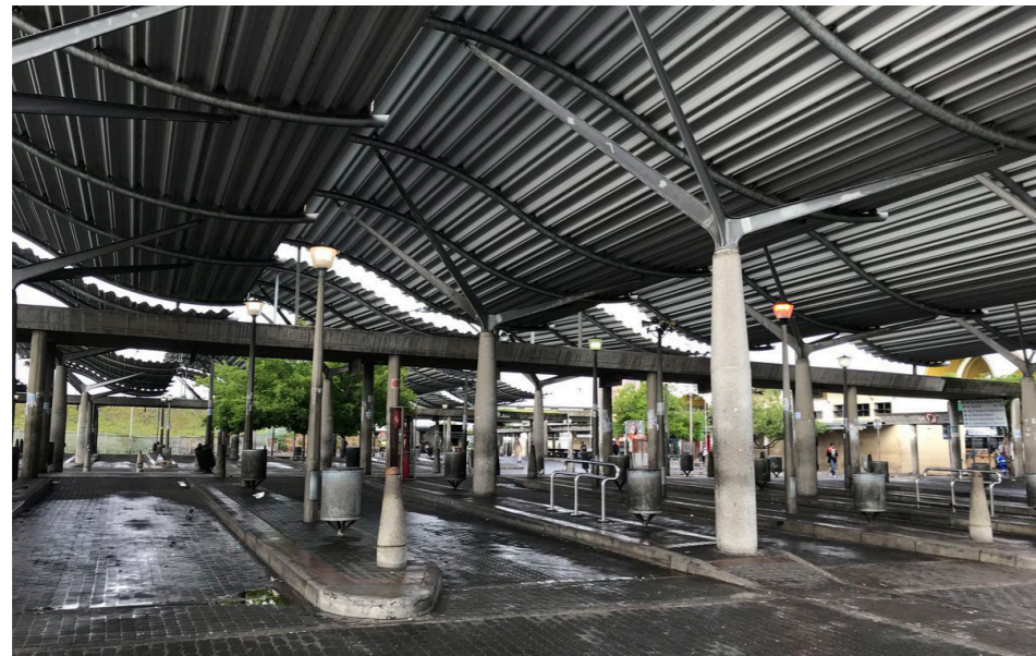
Figure 5.11 Curved, corrugated metal roof sheeting shading structures (EWN 2018).
