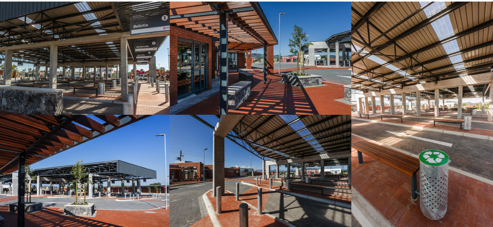
Figure 5.43-5.48 The taxi rank comprises a 10-lane taxi loading area with several naturally lit, sheltered and open waiting areas with a diverse range of robust, accessible, and comfortable seating options (SVA International 2021).
