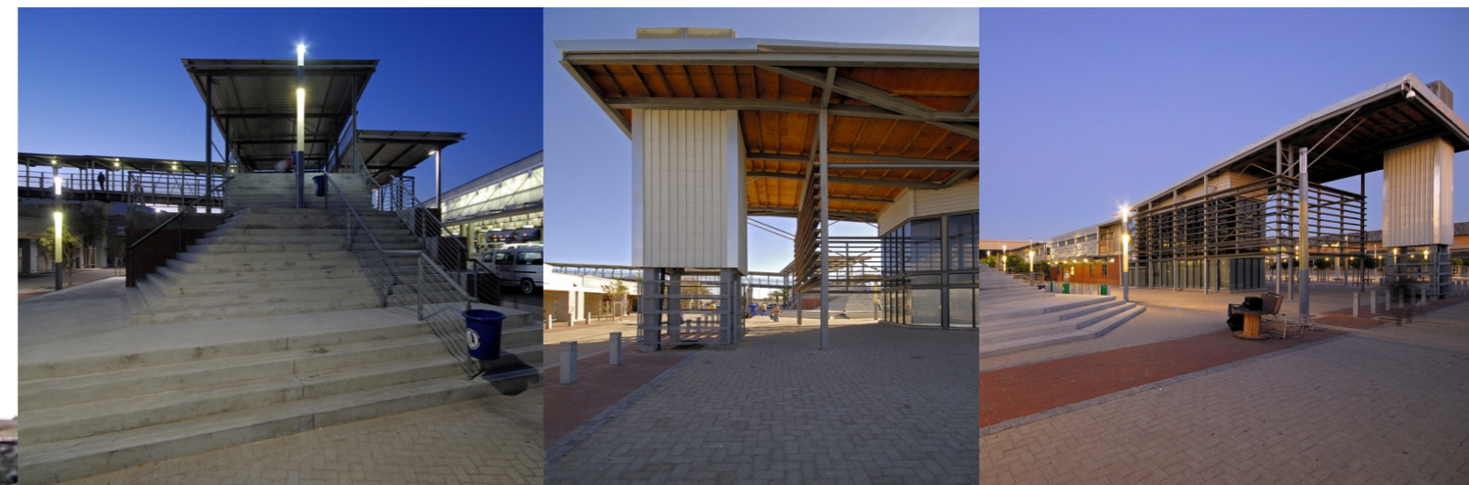
Figure 5.30-5.32 The tectonic modular bus and taxi shelters, designed in such a way as to provide protection to commuters during harsh summer and winter climatic conditions (Artefacts 2002).
