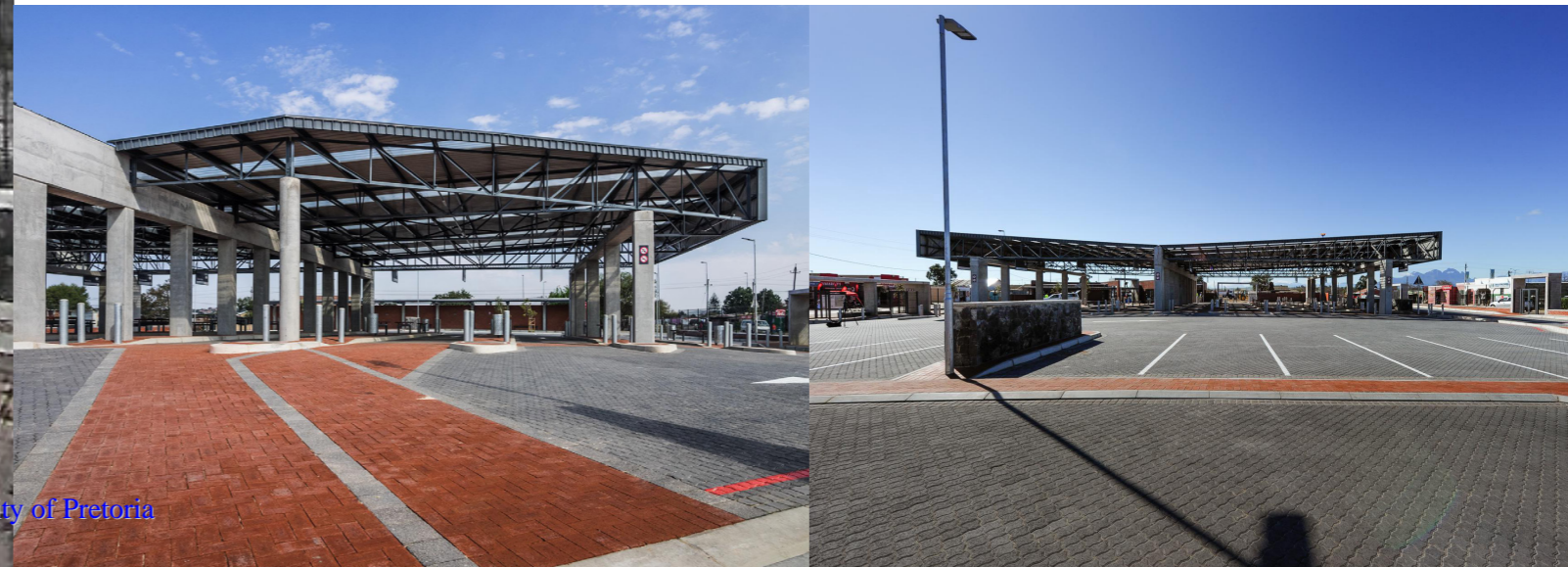
Figure 5.41-5.42 The considerable roof area is effectively utilised to collect rainwater as well as the inclusion of a 20kVA photovoltaic assembly system with battery back-up (SVA International 2021).
