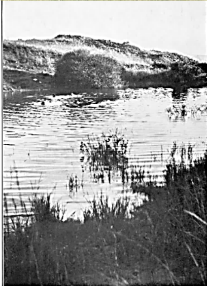
Figure 271. Water accumulation on site (Author 2021) Figure 272. Dam on site before 1910 (Hansen 2016)
