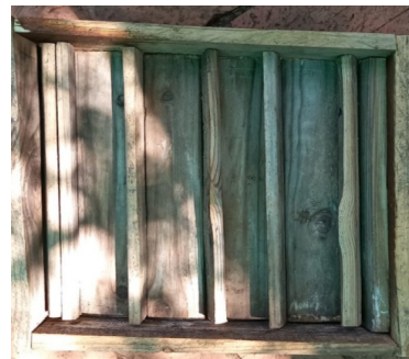
Combustible material – planks
