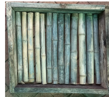
Combustible material – reed lathes
