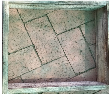
Timbre formwork – 400 x 400 blocks
