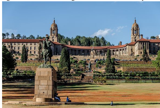
Figure 3. Photograph of the bad condition of the southern lawn of the Union Buildings (Richman 2016)
