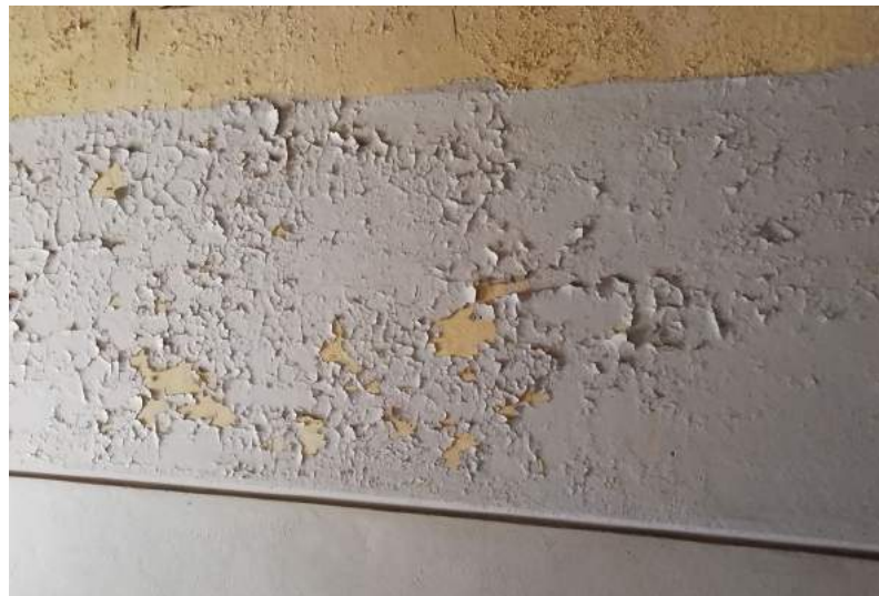
Fig.91: (Left) Surface of the exterior skin of the Capitol theatre: unarticulated and in a state of decay (Author 2021).
