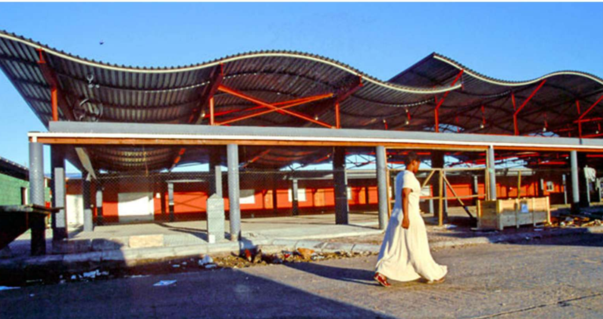
Figure 2.25: Gugulethu Central Meat Market Plan (Carin Smuts Architects 2021) Figure 2.26: Gugulethu Central Meat Market Perspectives (Carin Smuts Architects 2021) Figure 2.27: Landmark, Permeability, Flexibility Diagrams (Author 2021)
