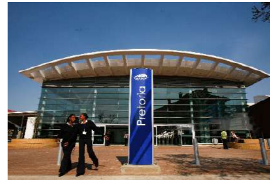
Figure 3.12 View of Pretoria Gautrain station main entrance (Bloomberg 2011)
