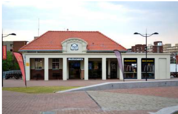
Figure 3.10 Photo of Old Audit building - elevation toward forecourt (Author 2021)
