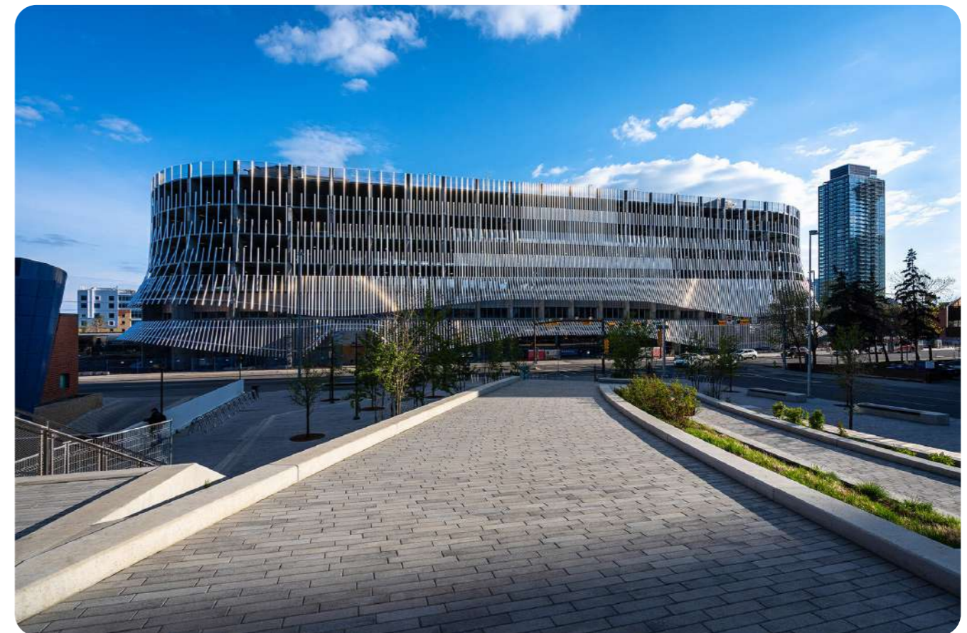
Figure 7.3 Platform innovation centre + parkade on 9 th Avenue, Calgary (Calgary Municipal Land Corporation 2020)
