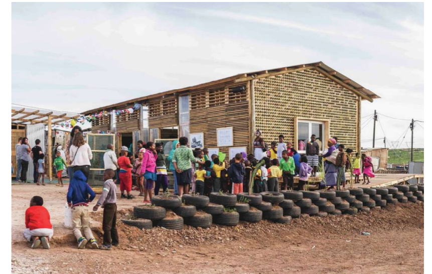
Figure 3.22. Silindokuhle community hall (Loots 2015)
