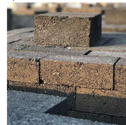
Figure 5.19. Plastic bricks (Ramtsilo 2018)
