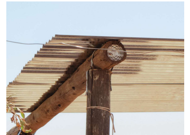
Figure 5.6. Dwelling roof structure (Author 2021)
