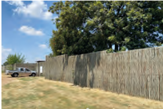
Wattle screen of public swimming pool
