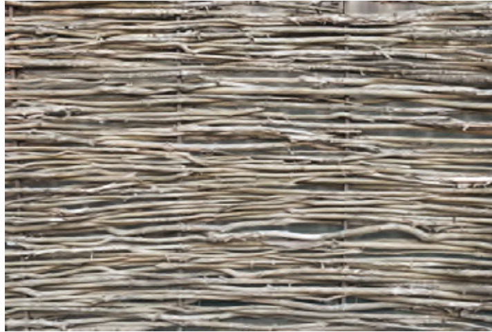
Fig 147: Wattle ceiling and screen (Solid earth 2021).
