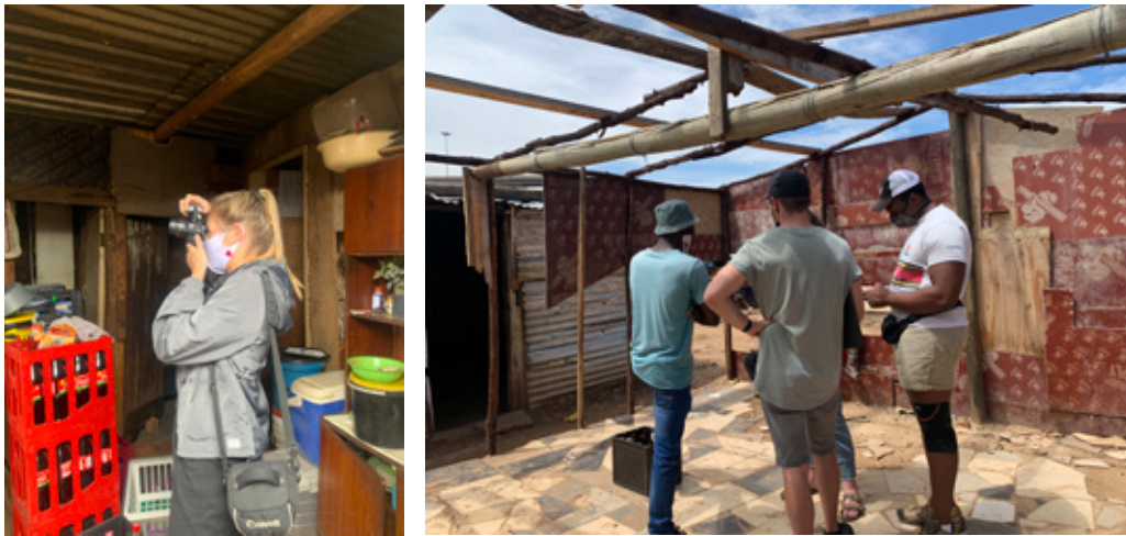
Figure 6.9: The liberal use of timber elements used for structural and cladding purposes (MPIP 2021).
