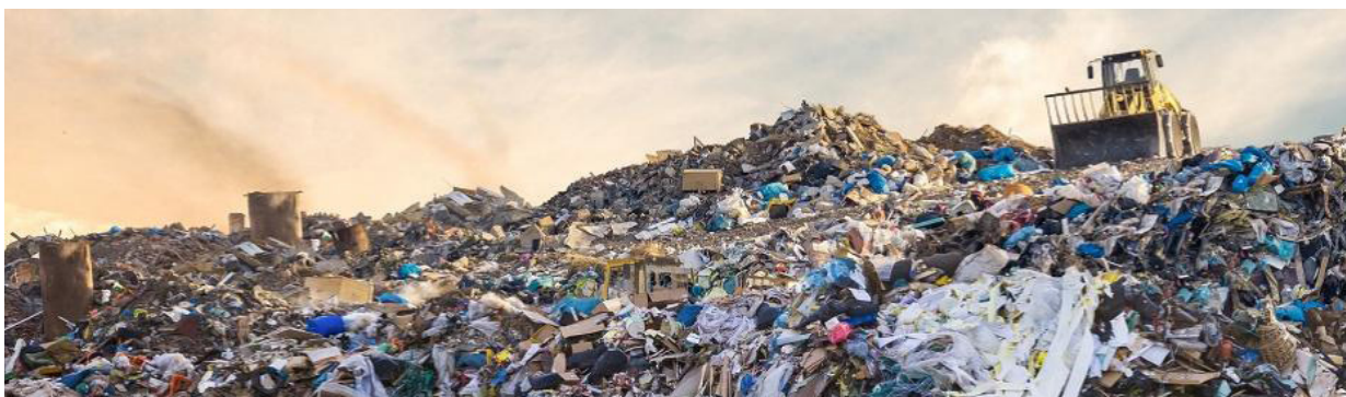
Fig. 1.3: Typical South African landfill dealing with environmental protection issues and holding capacity (DTE 2019).
