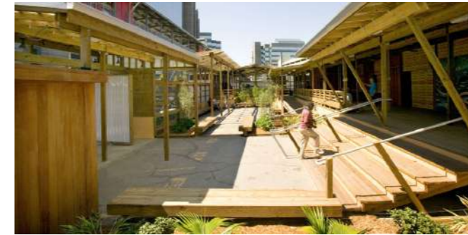
10.8. Photo of St. Joseph Rebuild Centre (Farbstein et al. 2009).
