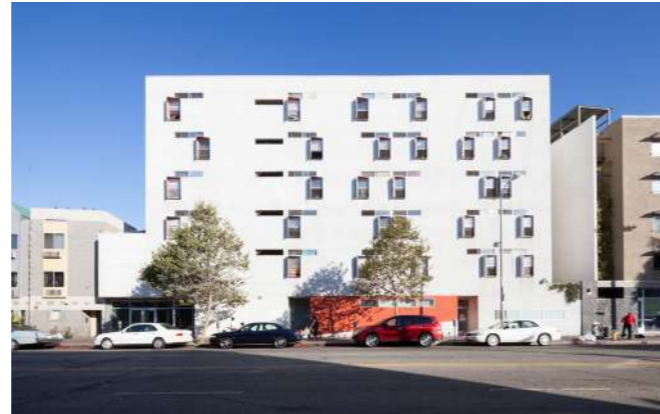
14.3. Photograph of southern (street) elevation (Maltzan 2020).
