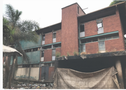
1960s/70s Hostel Building: Functional Regionalist / International Style
