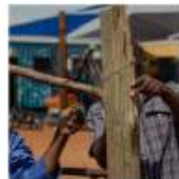
Through practical application and previous experience a fence is built from materials found on site.
