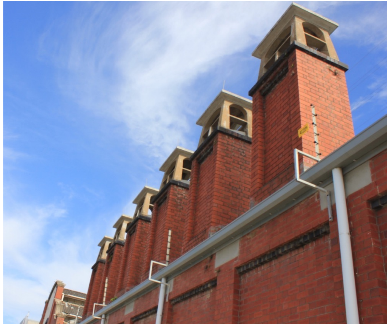
Figure 119: Chimneys on site signifying cooking (Author 2021)
