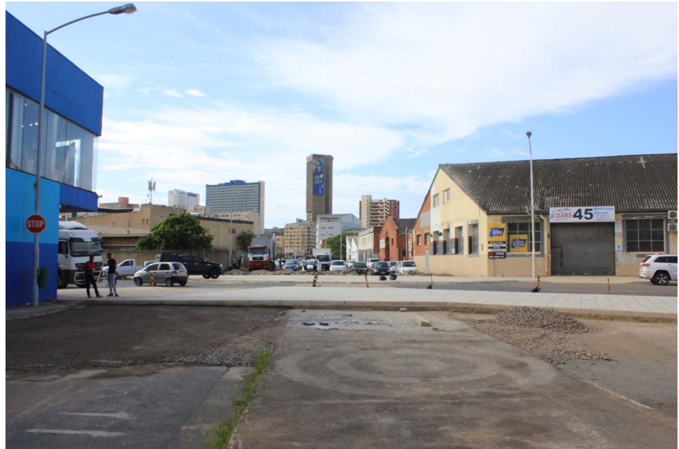
Figure 31: Existing covered canal (Author 2021)
