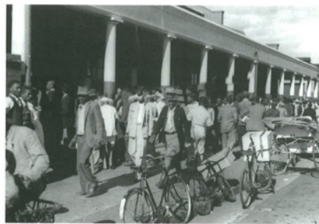
Figure 17: Beer Hall street facade, (AMAFA Report 2015: 7)
