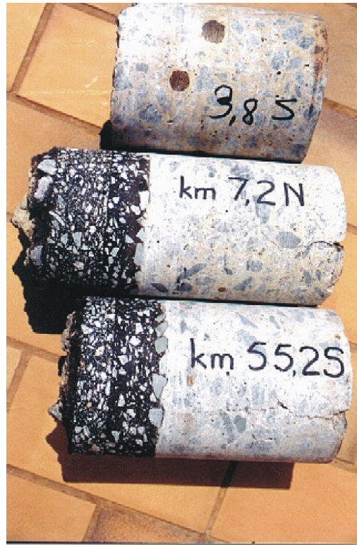
Photo 4: Good adhesion between asphalt and concrete
