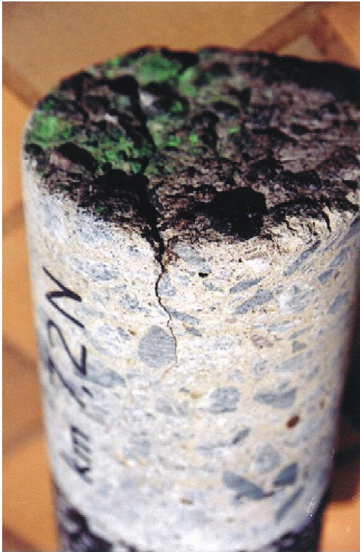
Photo 1: km 7,2 N - Surface weathering due to high slag content
