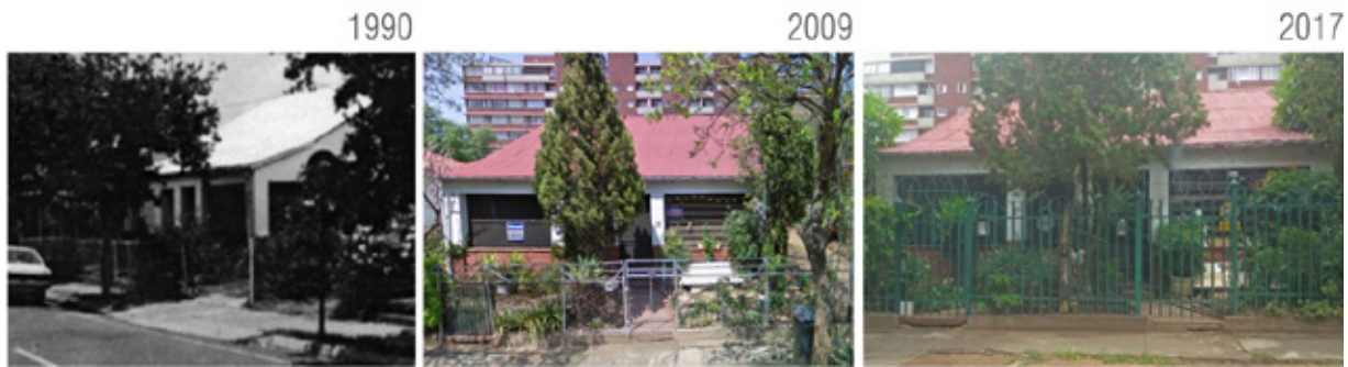
Figures 5.1 to 5.3: 15 Tulleken Street (1990) (Le Roux 1990: 160), 15 Tulleken Street (2009) (Google Earth 2017) and 15 Tulleken Street (2017) (Brümmer 2017: 26).
