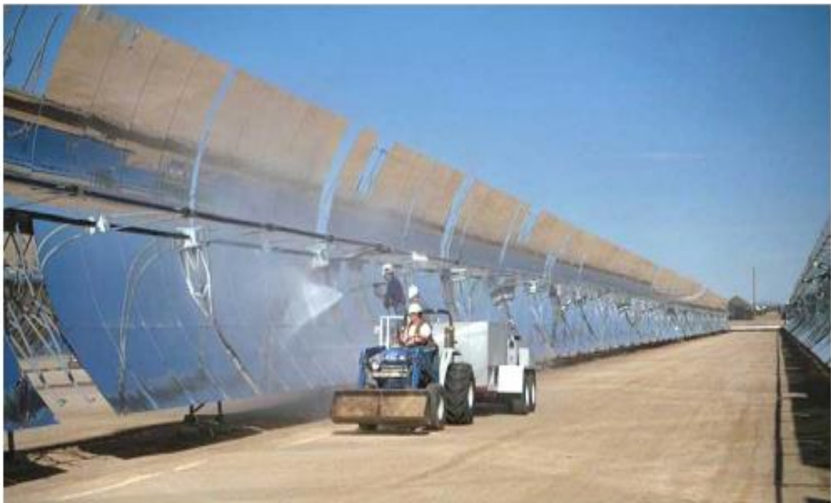
Figure 2.11. High-pressure cleaning with hand-held nozzle (Source: Cohen, et al., 1999)
