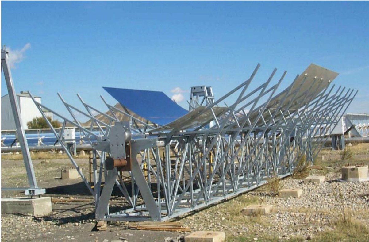
Figure 2.7. Bearing structure of a PTC (Source: Günther, et al., 2010)
