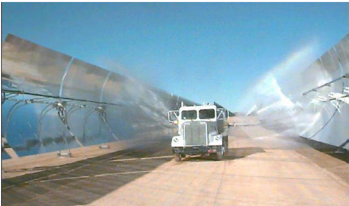
Figure 2.13. Simultaneous cleaning of the mirrors with a "deluge-type" stream (Source: Cohen, et al., 1999)
