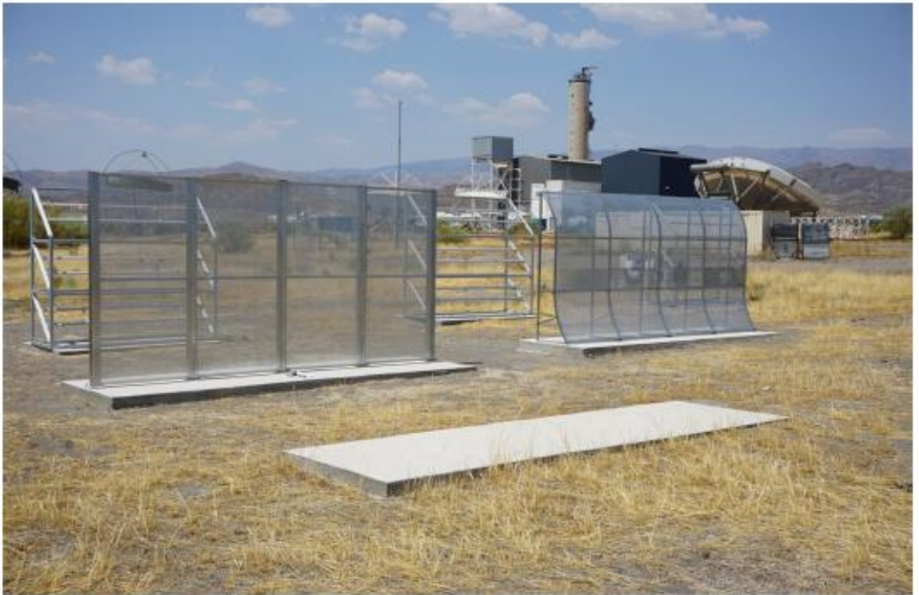
Figure 2.19. A wind barrier structure (Source: Bouaddi, et al.,2018)
