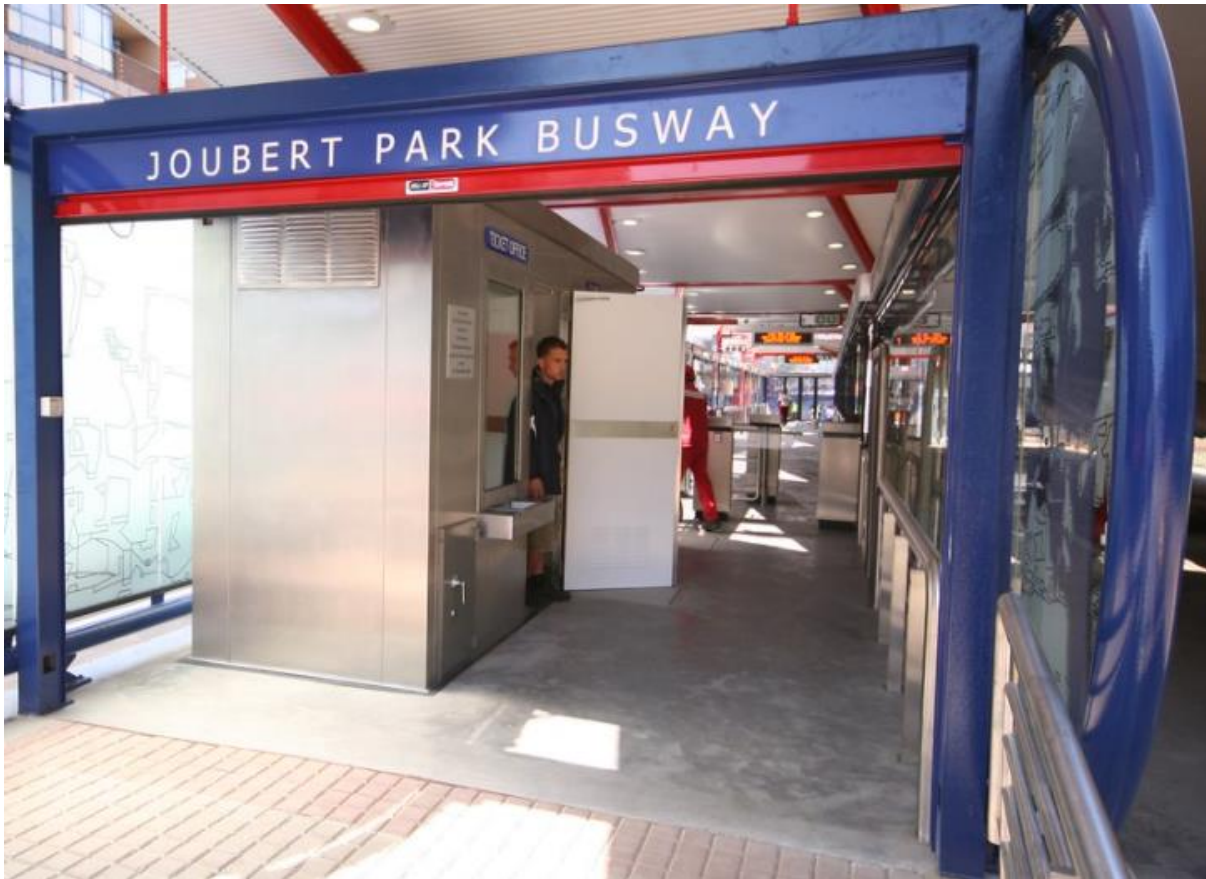
Figure 4:26 Entry and exit point at Joubert Park Station
