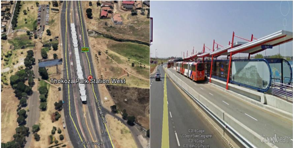
Figure 4:18 Thokoza Park BRT Station in Soweto (Source: Google Earth)
