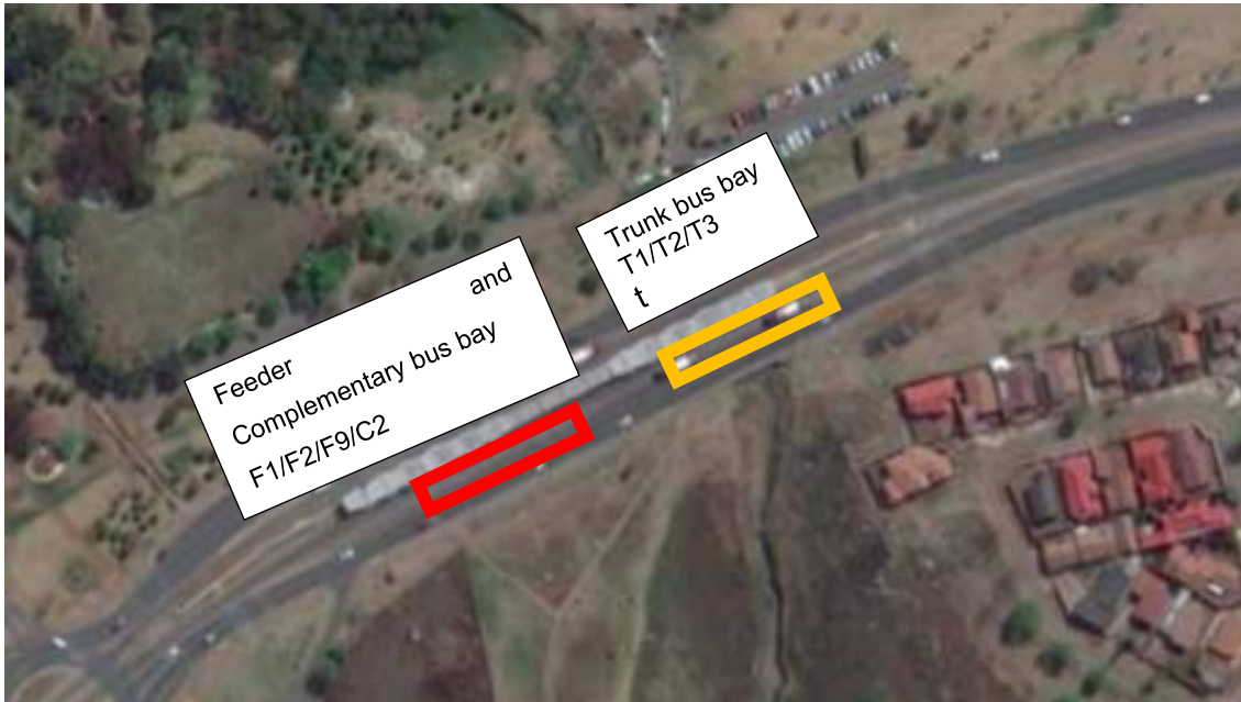
Figure 4:17 Docking station for trunk, feeder, and complementary buses at Thokoza Park Station
