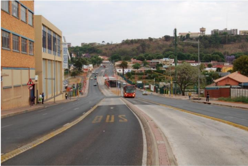
Figure 4:10 Median bus lanes for BRT in Johannesburg
