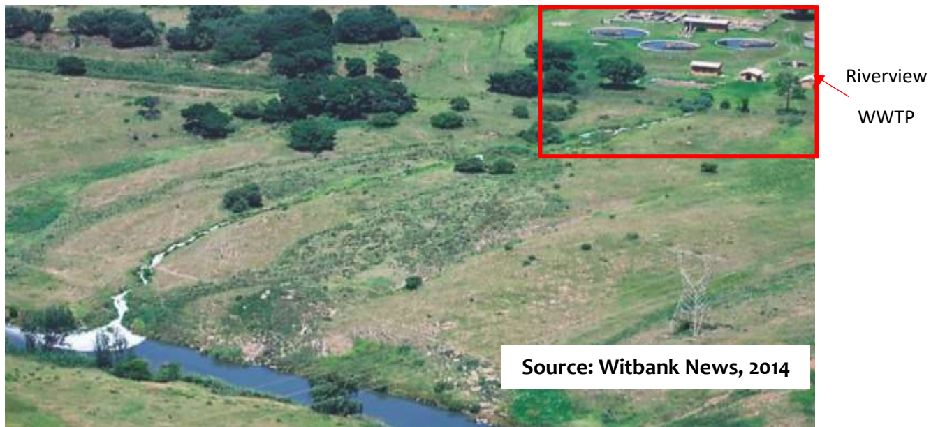
Figure 7: This is a picture regularly seen, white foam coming from Riverview Wastewater Treatment plant and running into Olifants River.
