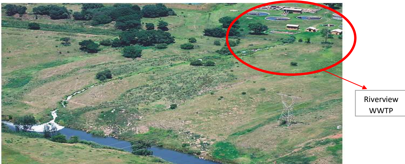
Figure 17 : This is a picture regularly seen, white foam coming from Riverview wastewater treatment works and running into Olifants River. (Witbank News, August 13, 2014)
