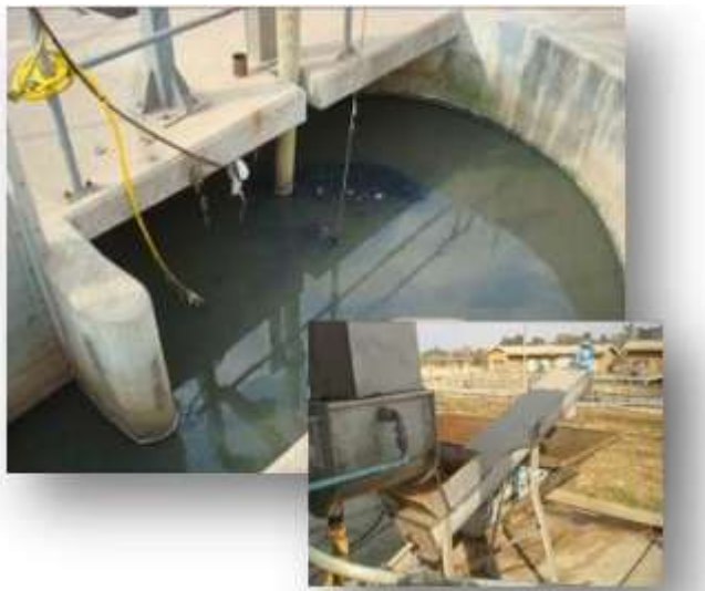
Figure 16: The condition of inlet area, Naauwpoort WWTP during 2010/2011 NGDA
