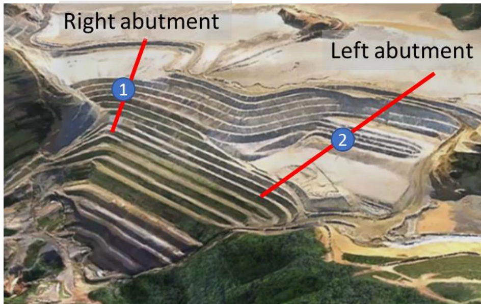
Figure 2.5: Location of the right and left abutments of the Fundão tailings dam, after Morgenstern et al. (2016)
