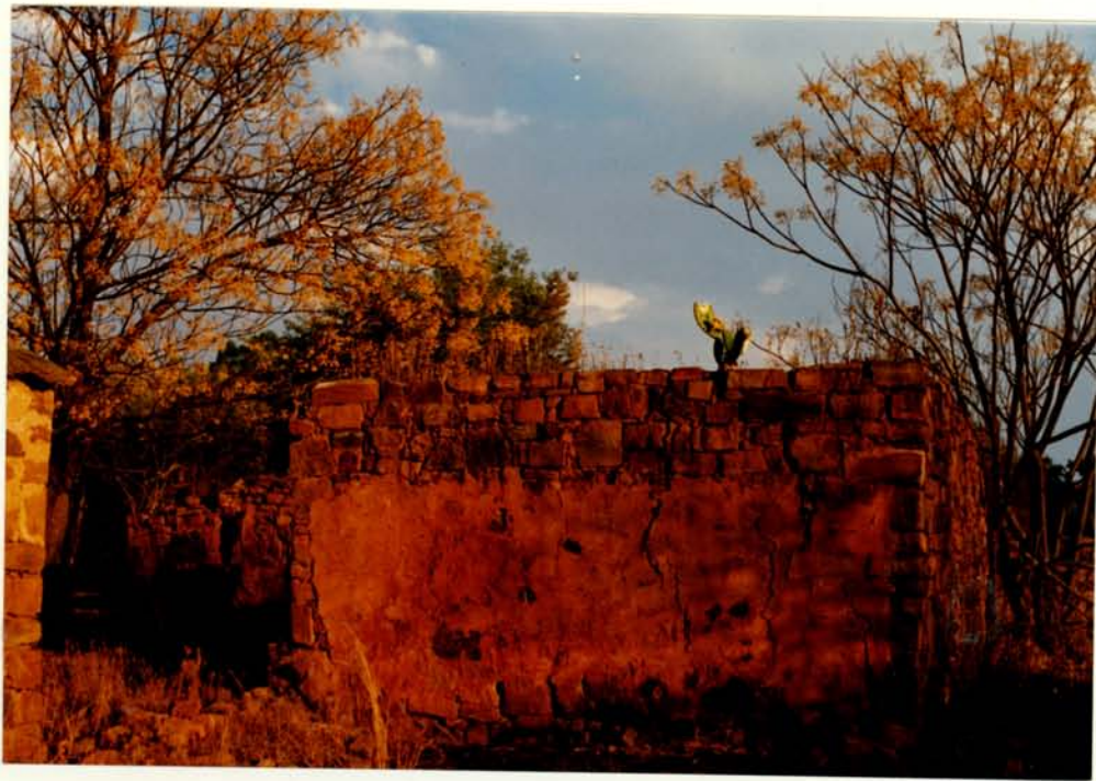
MUD PLASTER ON NORTH SIDE OF 11.24
