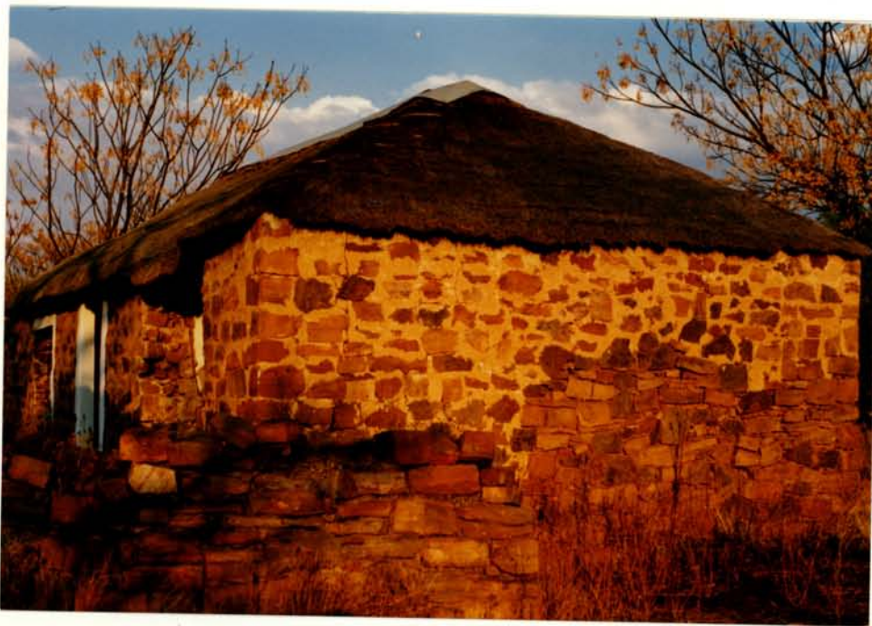
MORTAR FILLED JOINTS, THATCHED ROOF WITH SHEET METAL CAPPING
