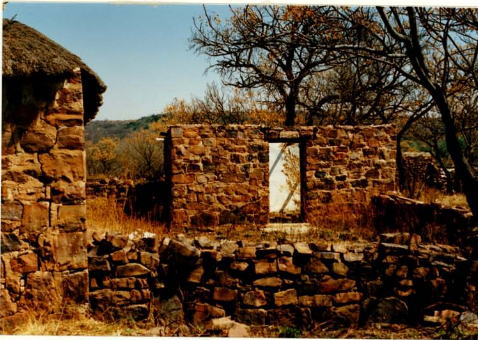
MORTAR FILLED JOINTS OF BUILDING CONTRAST WITH THOSE OF GARDEN WALL
