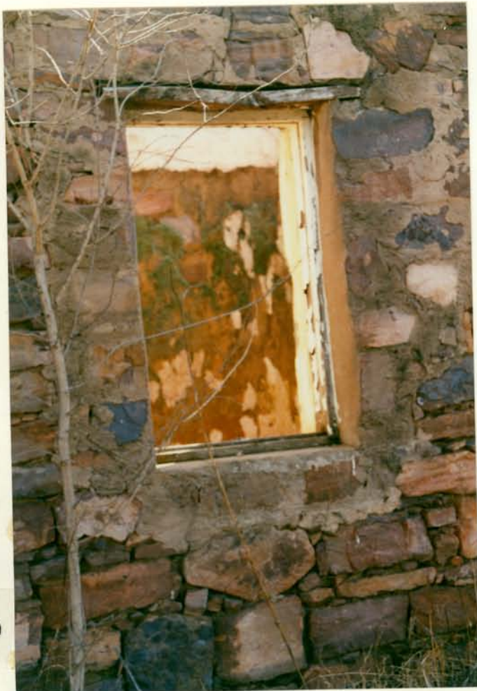
10. WINDOW IN SOUTH ELEVATION OF 11.28.
