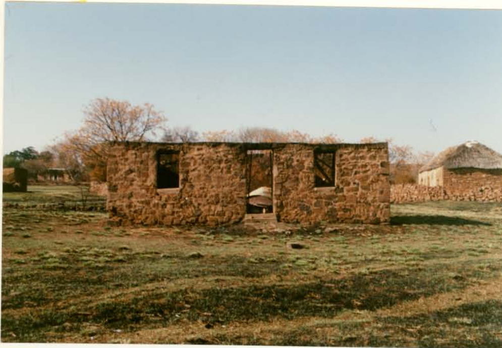
2. NORTH ELEVATION OF BUILDING 11.2.
