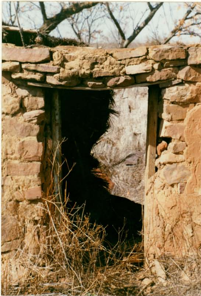
8. DETAIL OF DOOR
