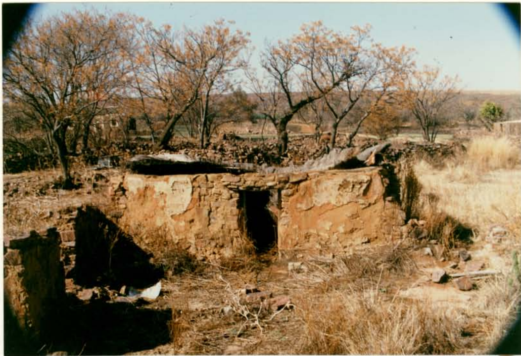
7. COW DUNG PLASTER CAN BE SEEN TO THE RIGHT OF THE DOOR OPENING ON THE NORTH FACADE OF 11.13.
