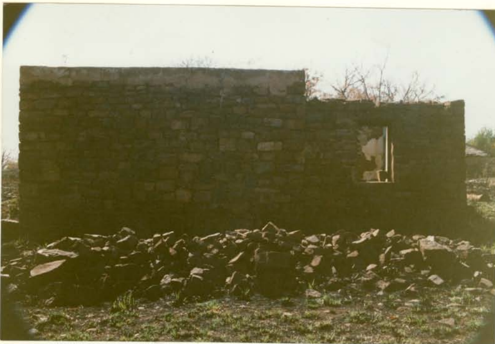
4. WEST ELEVATION OF BUILDING 11.28
