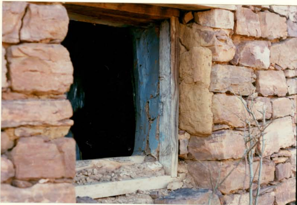
6. LEFT WINDOW ON EAST FACADE OF BUILDING 11.12
