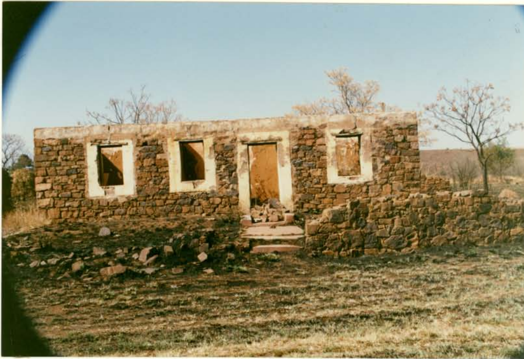
1. NORTH ELEVATION OF BUILDING 11.28
