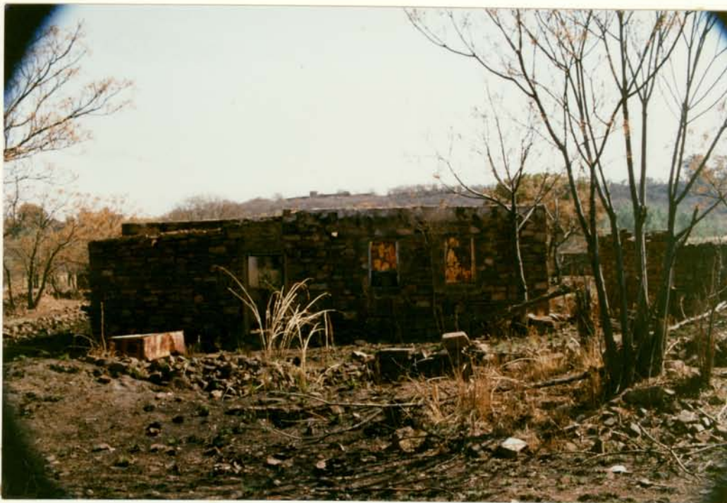
2. SOUTH ELEVATION OF BUILDING 11.28
