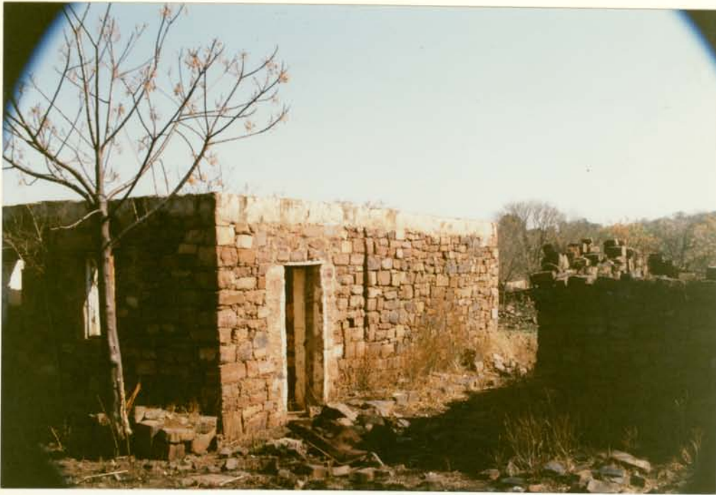
3. EAST ELEVATION OF BUILDING 11.28
