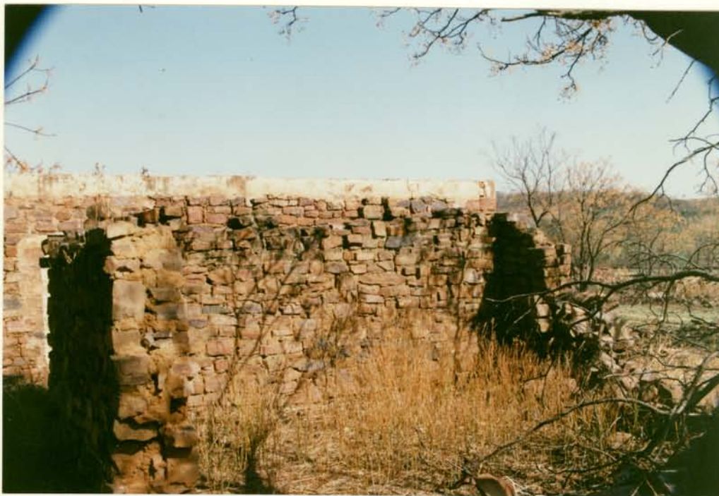
6. REMAINS OF BUILDING 11.27 TAKEN FROM EAST SIDE
