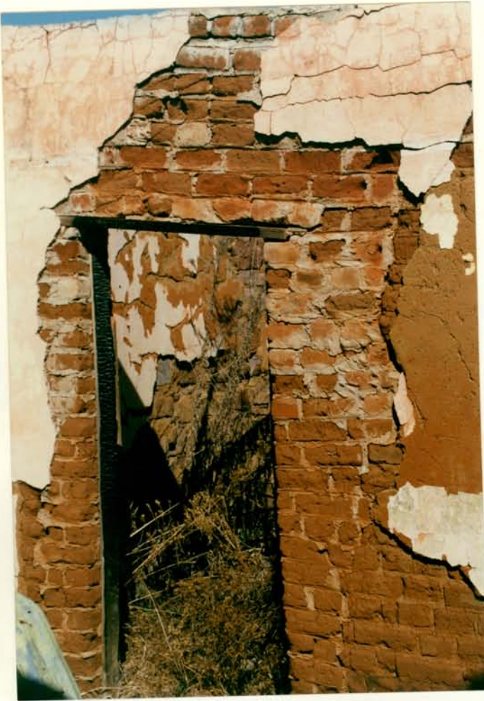
9. DOOR FRAME IN BRICK WALL OF 11.28.
