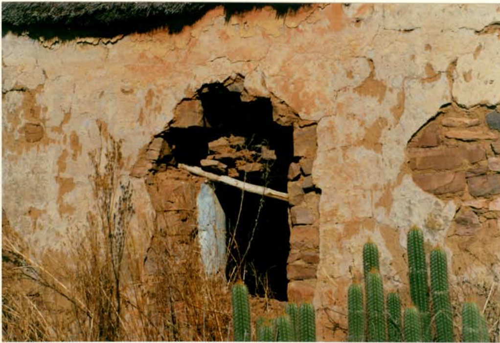
5. RIGHT WINDOW ON EAST FACADE OF BUILDING 11.12
