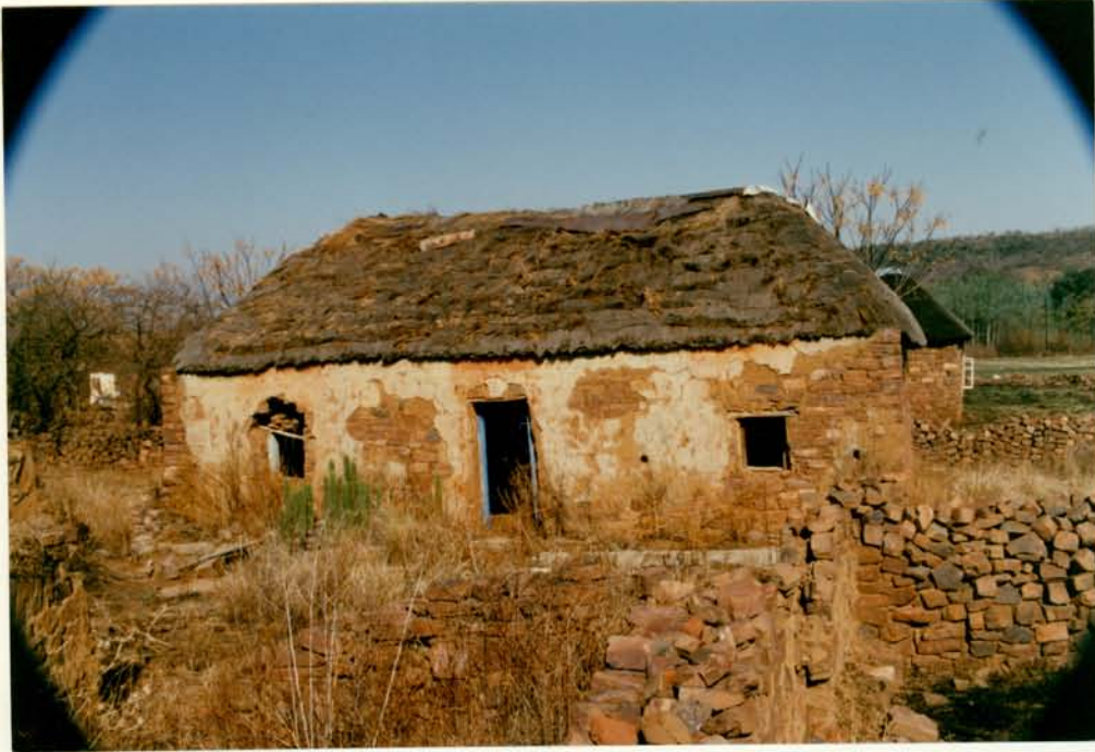
1. EAST ELEVATION OF BUILDING 11.12
