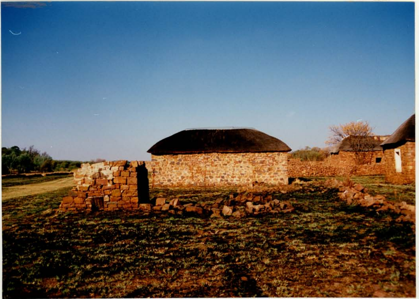
1. Building from the west with outbuilding and remains of garden wall
