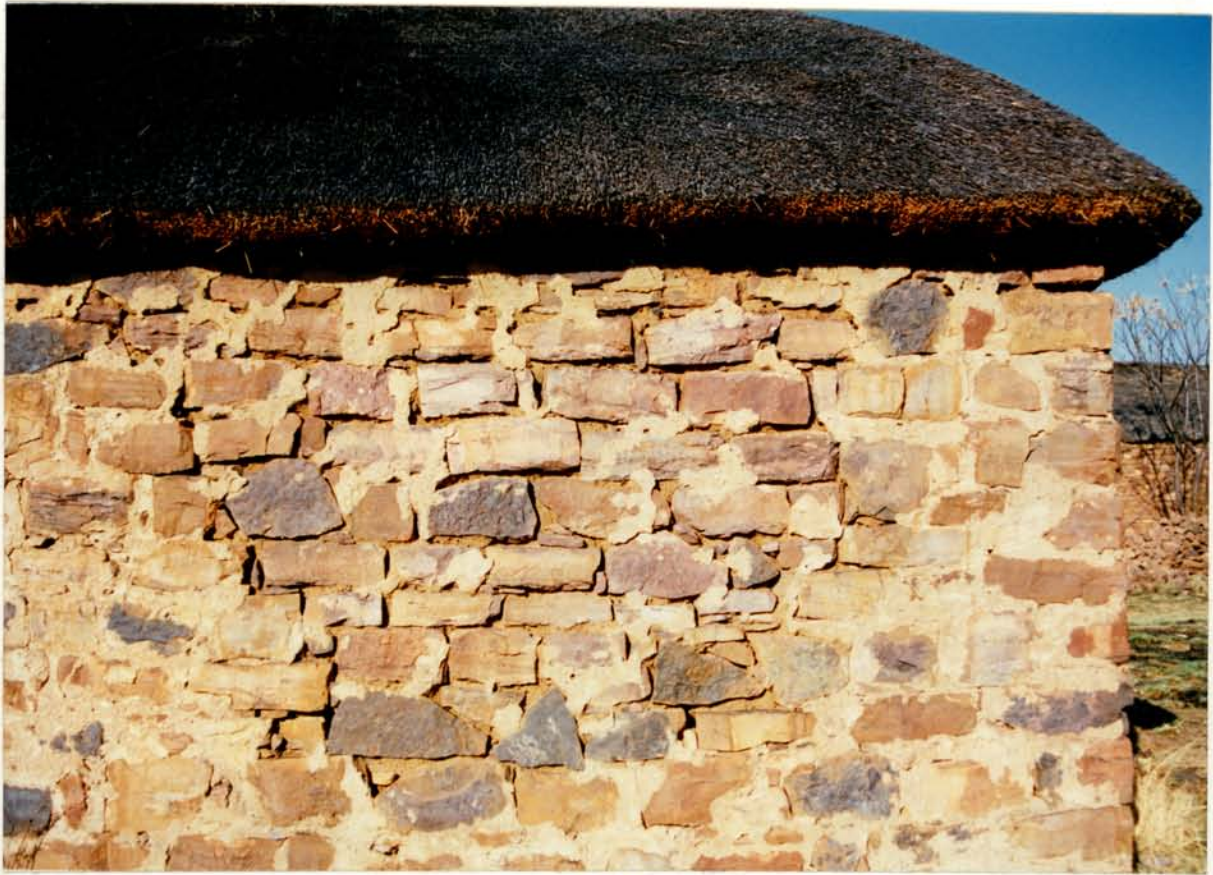
4. Former window (?) now closed up Western facade
