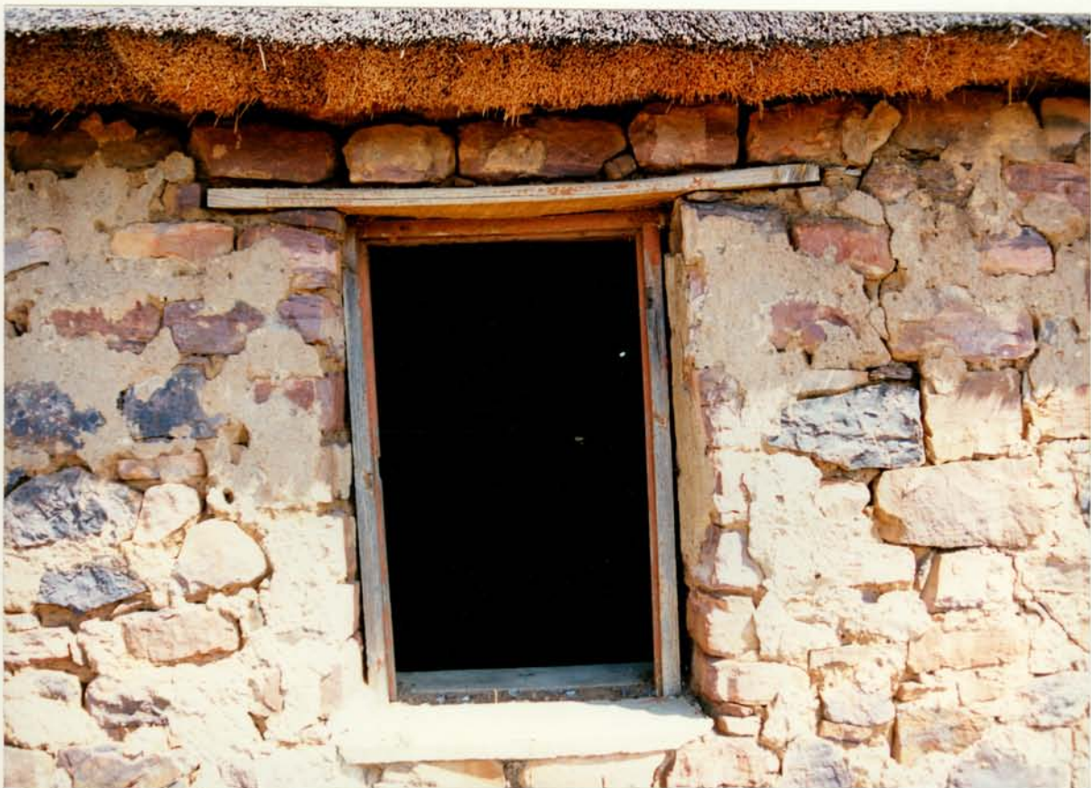
5. Window and lintol in northern room
