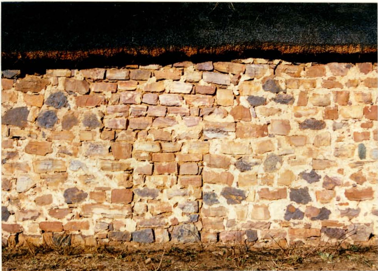
3. Closed door opening in western facade
