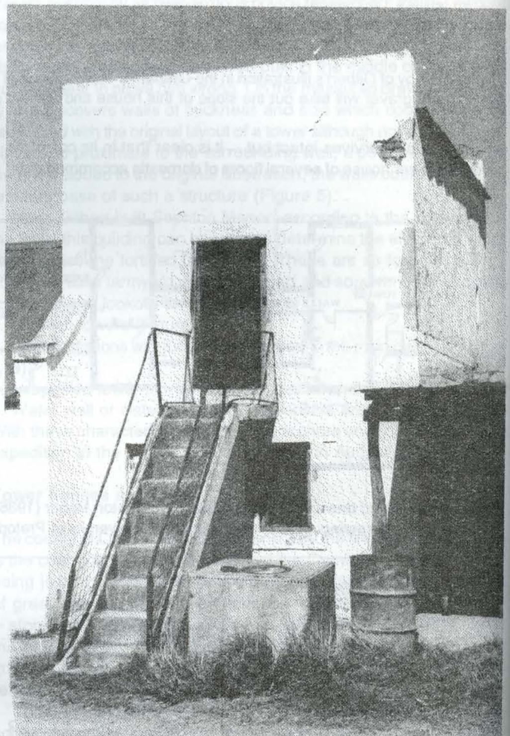
Figure 7 (Left) Tower in kraal wall as seen from outside. Note loophole at side of wall for raking fire. (Right) Tower from inside of Kraal. Note the stair to the upper storey and compare with that of the bastle house (see Figure 21).
