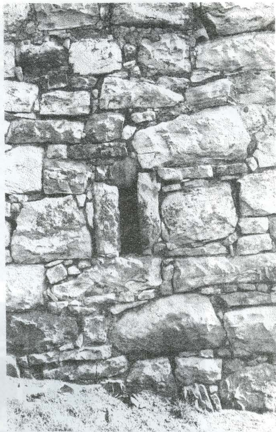
Figure 15 (left) Ventilation slot in the barn of Dean Farm, Cumbria, which might be mistaken for a loophole. (right) It however lacks the characteristic single stones at the broaching as shown by the Black Middens Bastle example.
