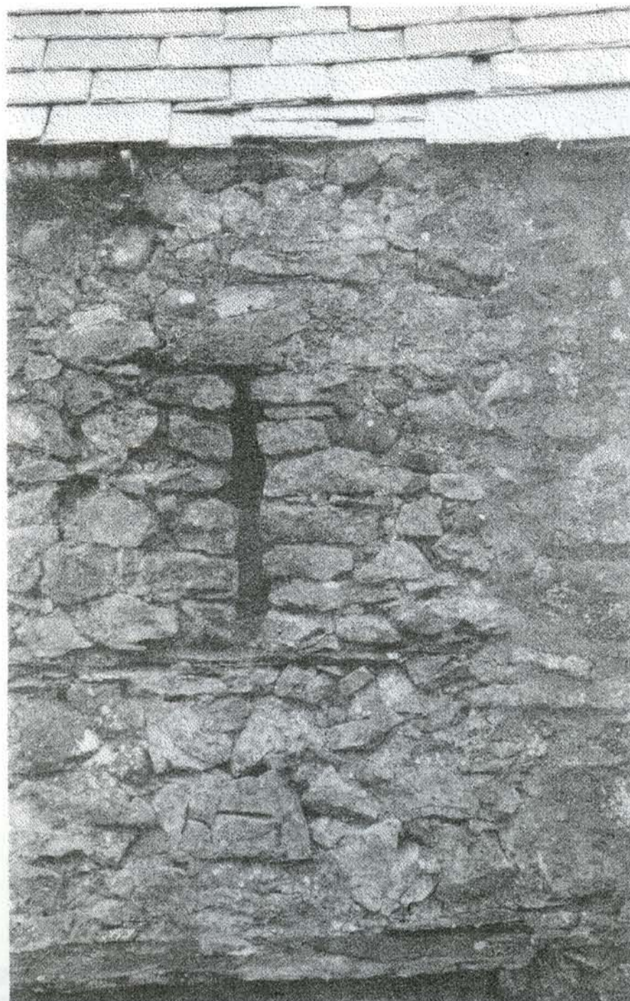
Figure 15 (left) Ventilation slot in the barn of Dean Farm, Cumbria, which might be mistaken for a loophole. (right) It however lacks the characteristic single stones at the broaching as shown by the Black Middens Bastle example.
