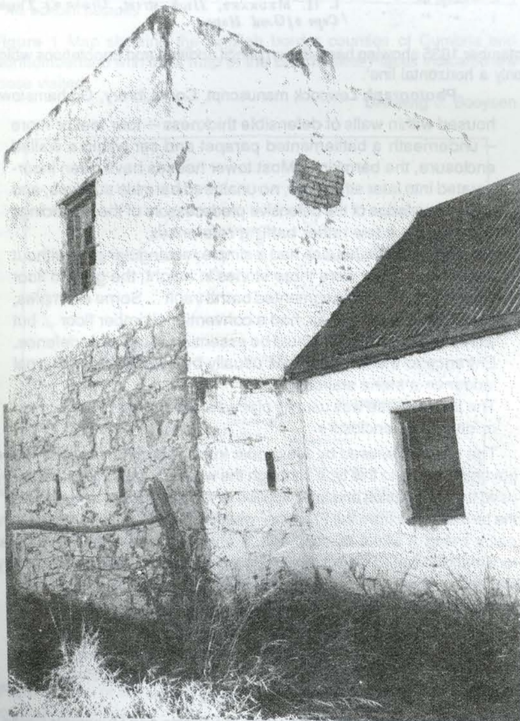
Figure 7 (Left) Tower in kraal wall as seen from outside. Note loophole at side of wall for raking fire. (Right) Tower from inside of Kraal. Note the stair to the upper storey and compare with that of the bastle house (see Figure 21).
