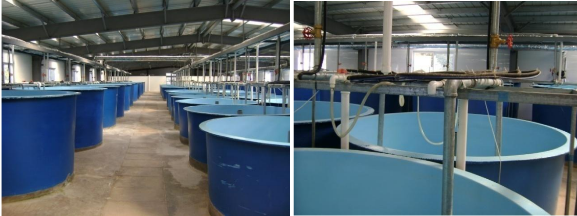
Figure 6 a. Hatchery tanks with big tanks on the left and small tanks on the right, b. blowers and pipe work into the tanks (Fraser, 2013)
