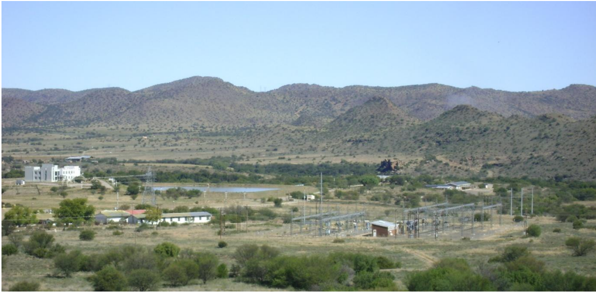
Figure 4. Overview of the setting and facilities at the demonstration centre (Fraser, 2013)
