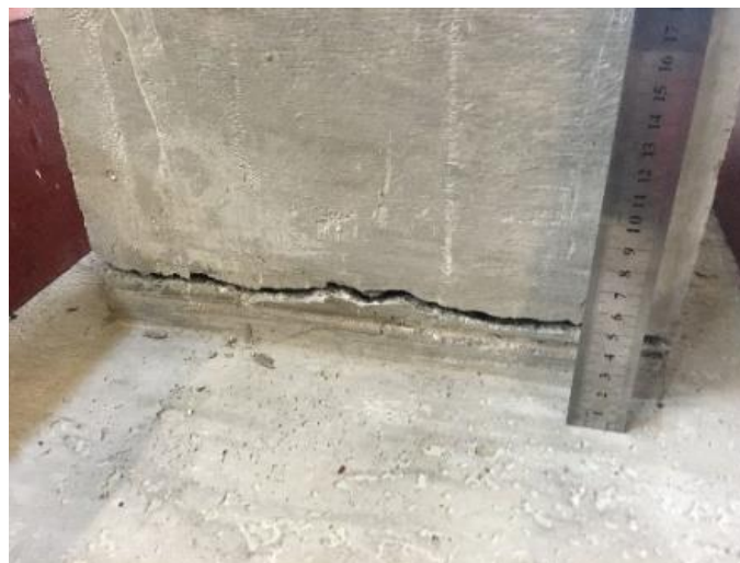
Figure 4-19 Cracking of concrete after the maximum acceleration had been applied to the footing during the El Centro earthquake at 0.68 g
