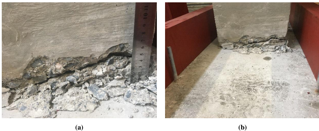
Figure 4-6 Cracking at the base of the reinforced concrete column during the cyclic load testing
