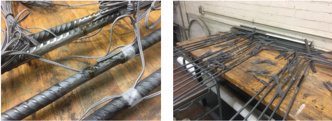
Figure 3-45 Strain gauge attachment to the reinforcing bars
