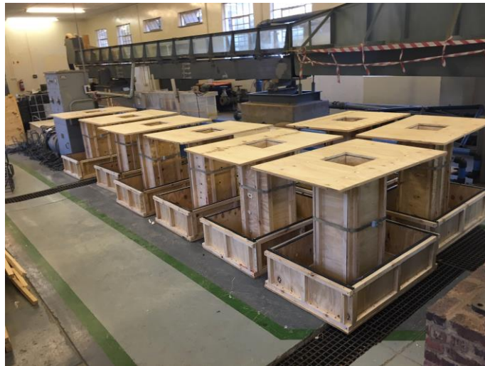
Figure 3-16 Reinforced concrete footing shuttering with base slab lid
