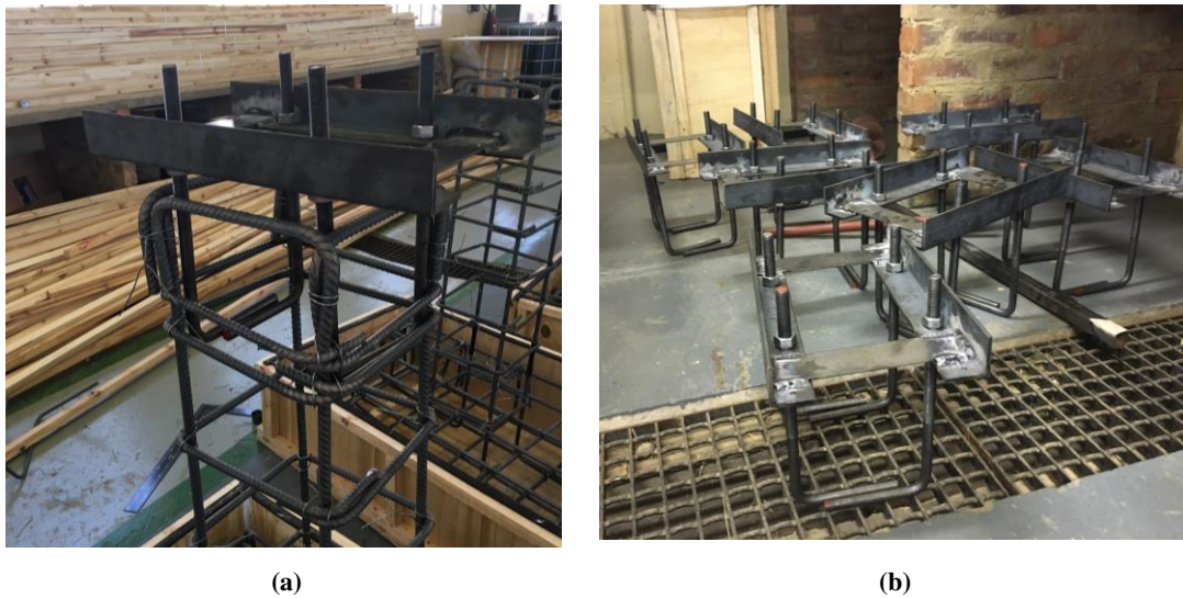
Figure 3-18 Holding down bolts and template
