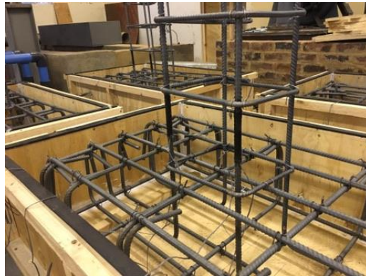
Figure 3-46 Strain gauges fixed to reinforcing bars
