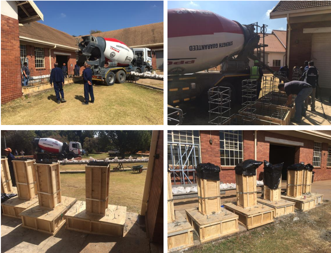
Figure 3-19 Concrete casting of the reinforced concrete footings
