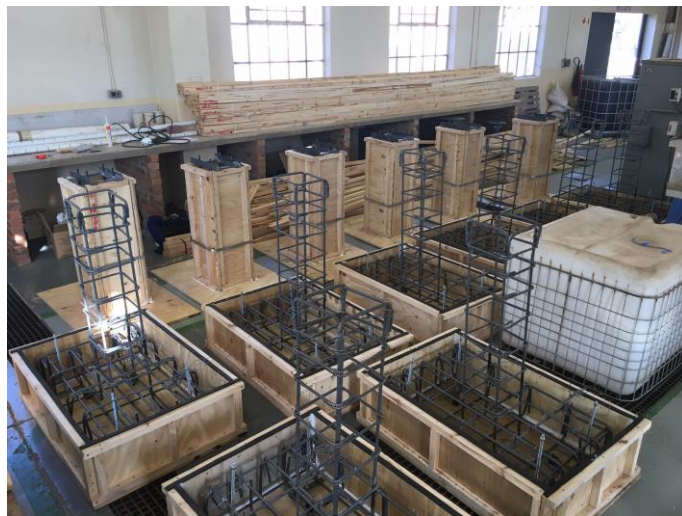
Figure 3-17 Reinforcement cages for the concrete footings
