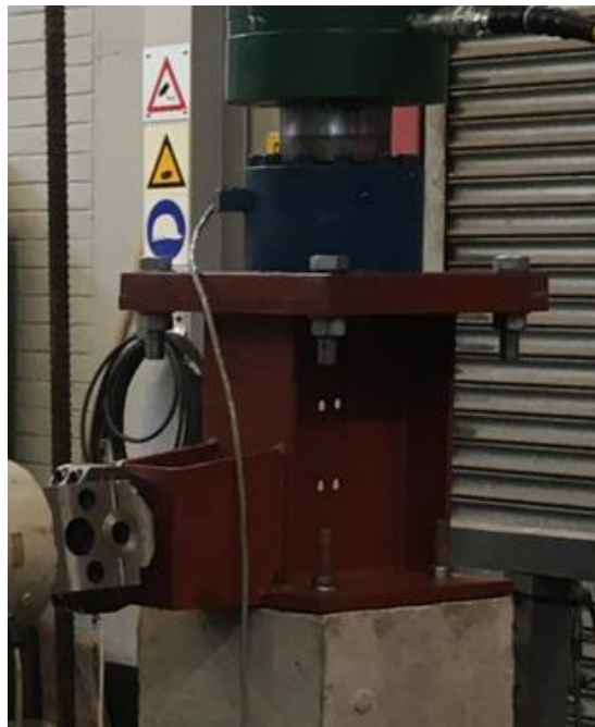
Figure 3-43 Steel actuator adaptor connection to the footing with the base plate and holding down bolts
