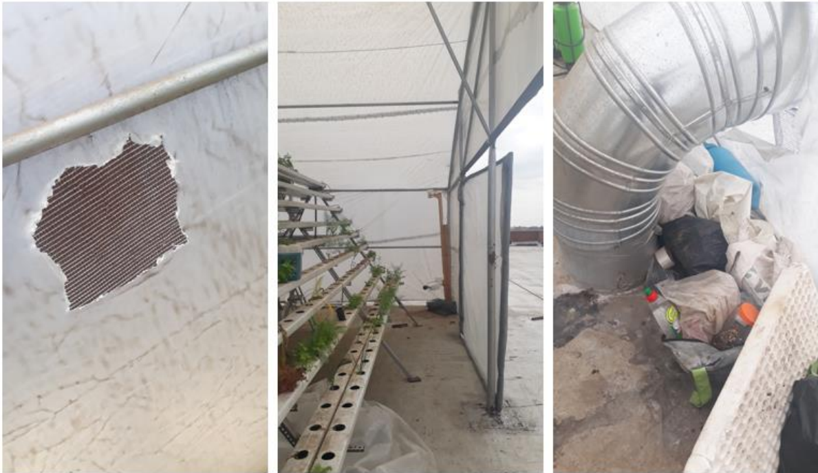
Figure 90: Envelope construction and finish. Photo taken at Stanop Building farm.
