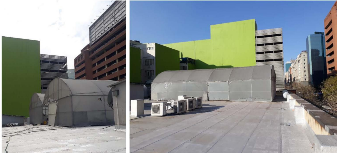
Figure 66: New Gate Mall Farm, Johannesburg.
