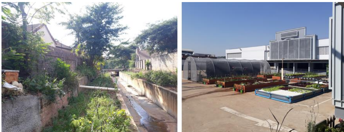
Figure 42: Retrofitting portions of infrastructure or parts of buildings. Location: South Africa.
