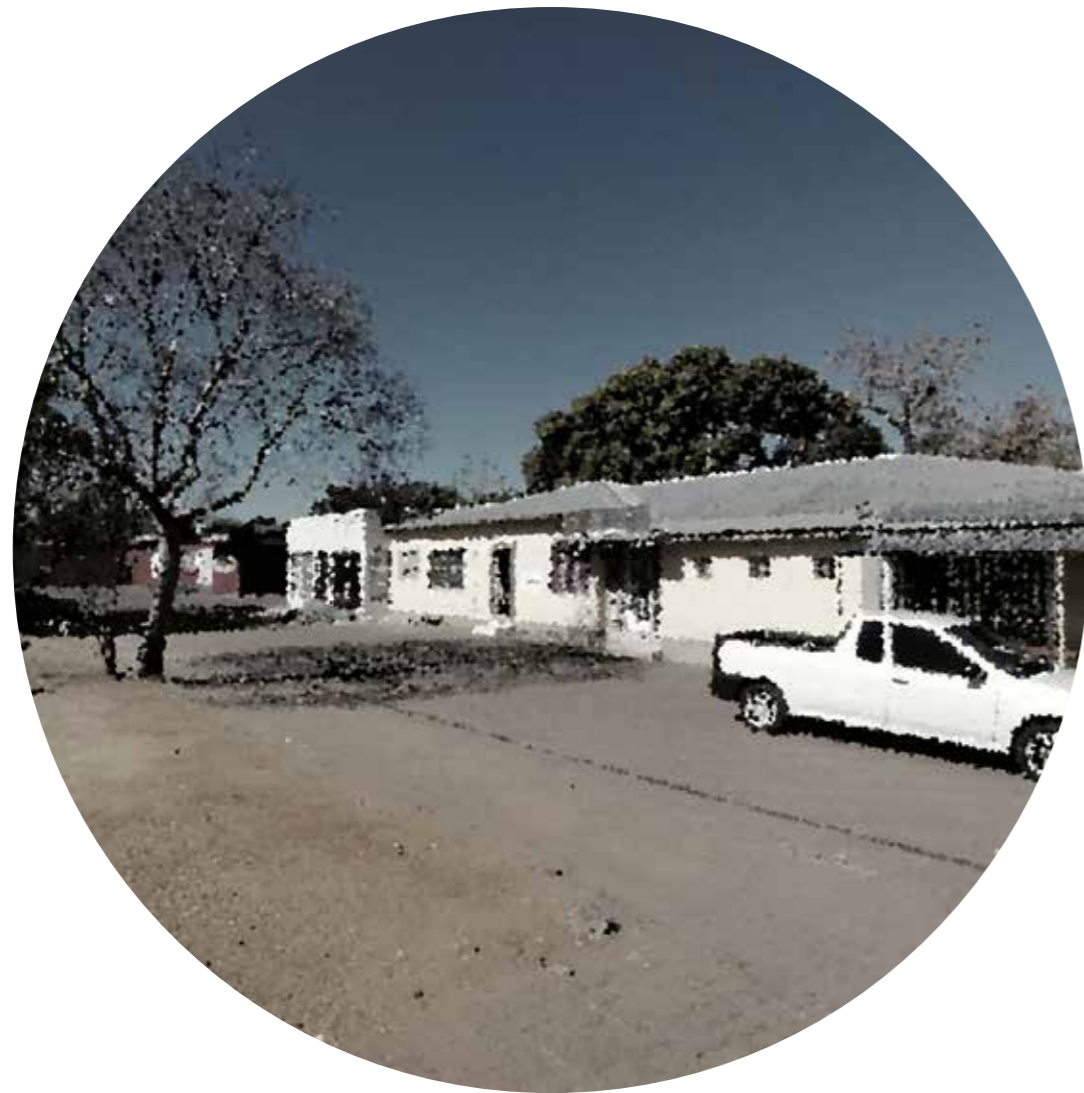
Figure 0.2: Derelict edge condition at site location where the brewery and cafe-bakery will be allocated (Author, 2020)
