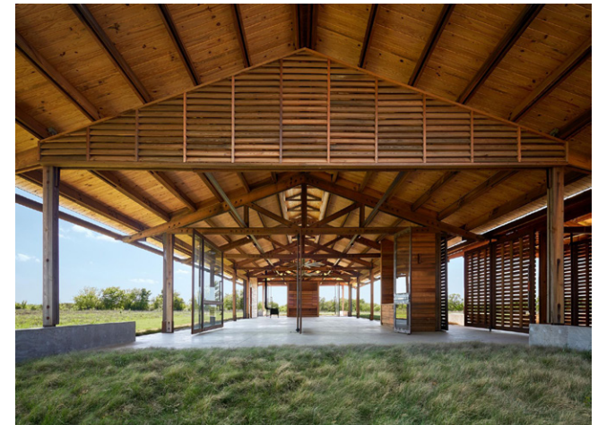
Figure82: Josey Pavillion (Lake Flato 2016)
