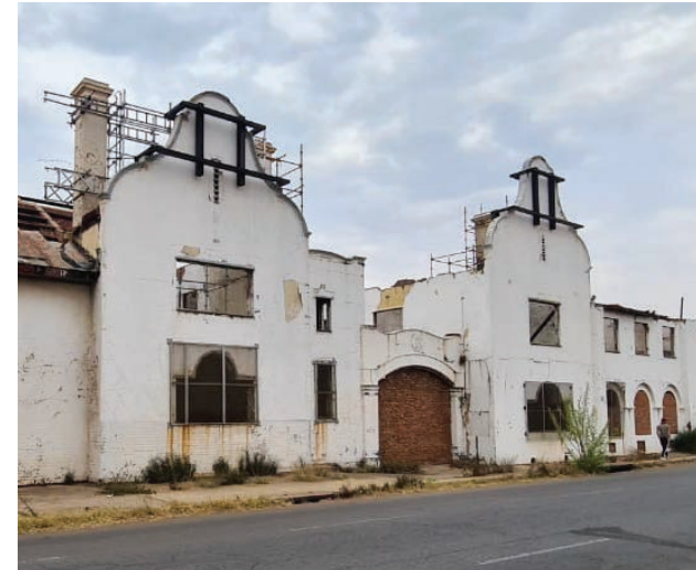
Building has already begun to be braced and structurally stabilised
