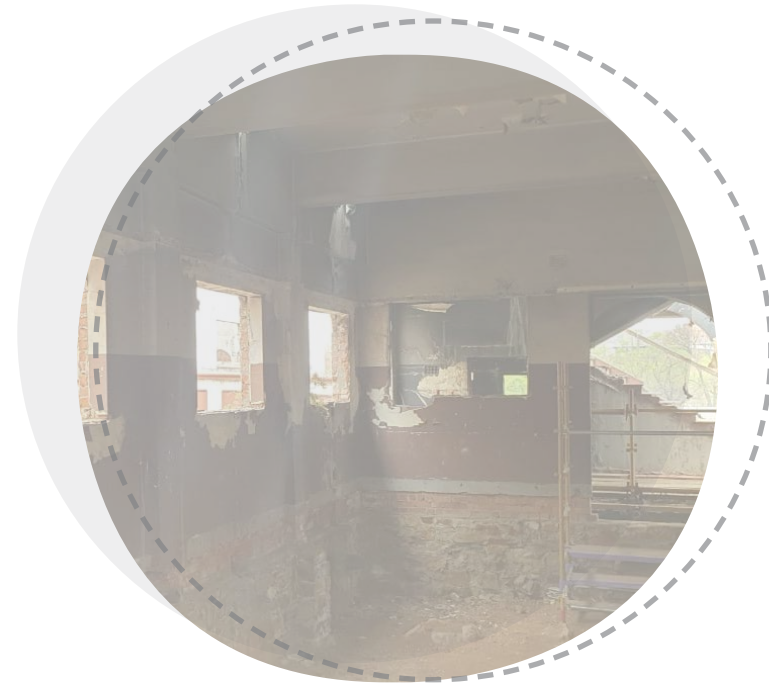
Figure 8.8. Interior View of Clubhouse (Author 2020)
