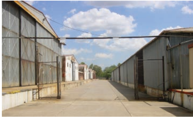
Figure 3.23. Left and Below. Military Health Base Depot at Thaba Tshwane (Jeremie Malan Architects 2020)
