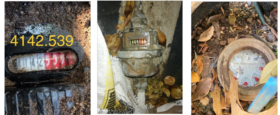
Figure 27: Examples of typical water meter reading captured during the water experiment (Author, 2020)
