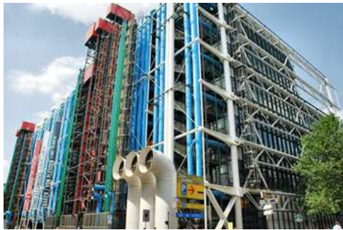
Figure 73: Pompidou Center (Potable water in pvc pipes is conventionally transported around a site and building under the ground and within the walls of a building in South Africa (Fennemore et. al., 2014). The ambition of exposing these otherwise hidden water sys
