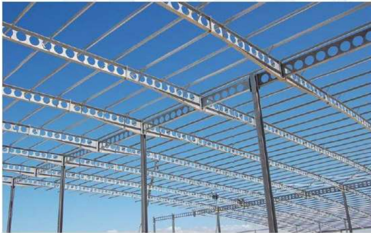
Figure 119: Cellular beams (Macsteel, 2019).
