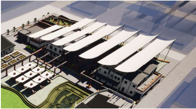
Figure 121: Stretched and pulled pvc membrane allows the roof to curve in all directions towards the central gutter (Author, 2020).
