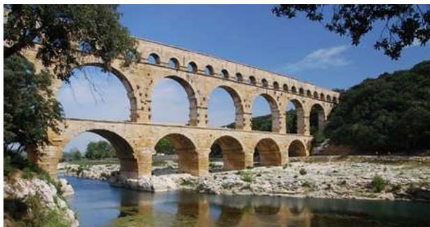
Figure 74: Roman aqueduct (Potable water in pvc pipes is conventionally transported around a site and building under the ground and within the walls of a building in South Africa (Fennemore et. al., 2014). The ambition of exposing these otherwise hidden water sys
