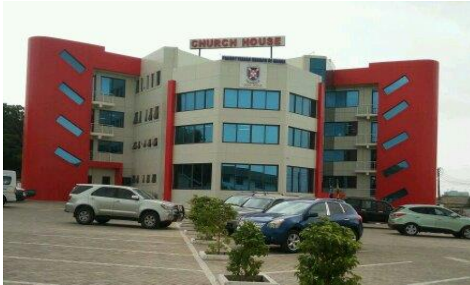
Diagram 2. The Headquarters of the Presbyterian Church of Ghana, at Kuku Hill, Osu, Accra.
