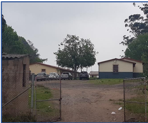
Photograph 4.1: School 10, KZN (24 October 2017)
